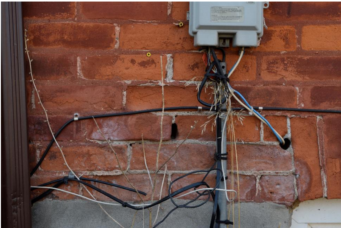
Image 32: Example of typical brick exfoliation resulting from poor water management.
