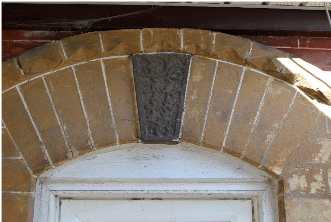
Image 17: Ribbon pointing present in voussoirs.
