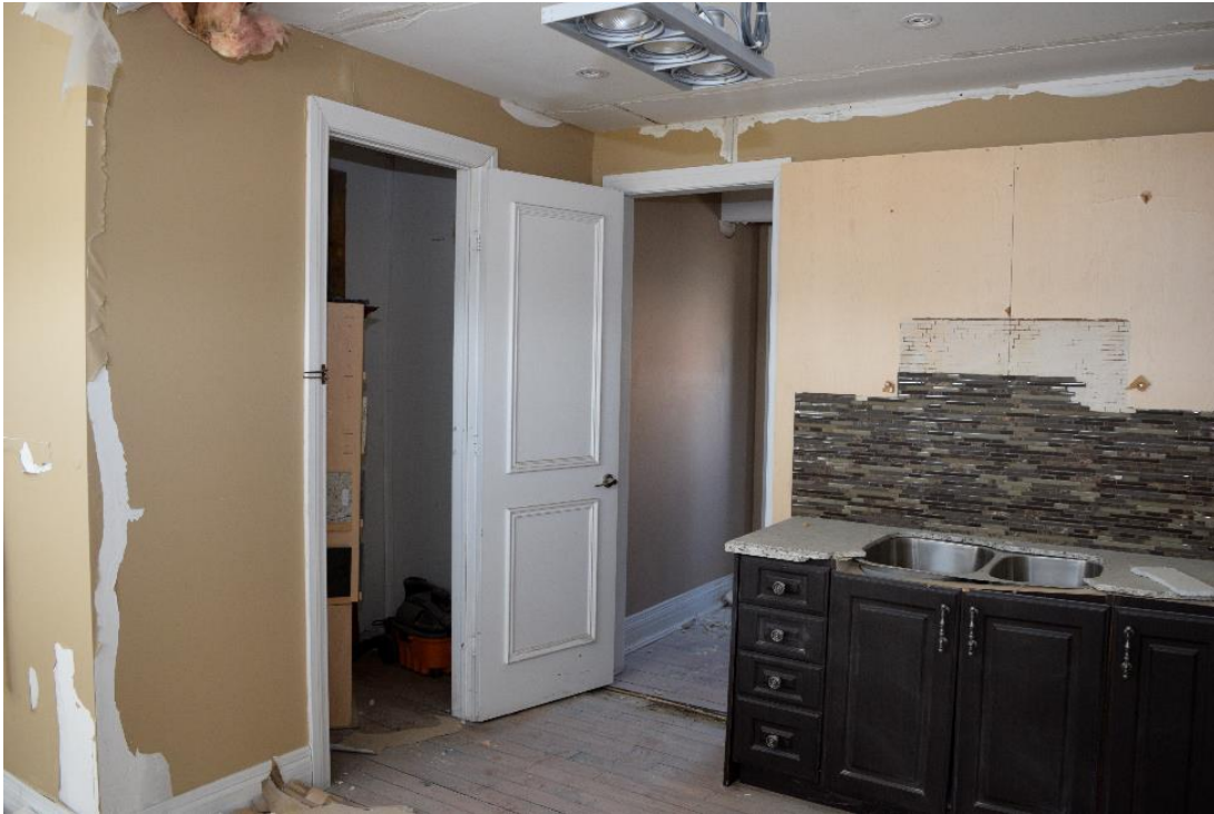
Image 39: Kitchen on first floor, facing southwest.
