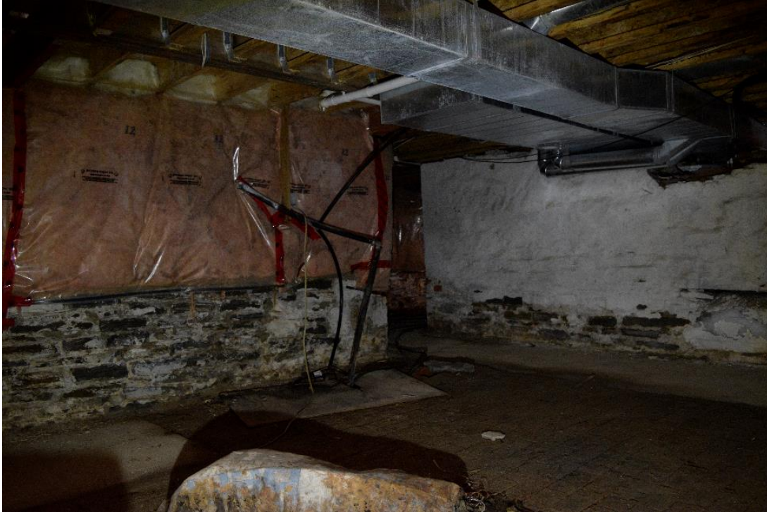
Image 53: Overview of basement.
