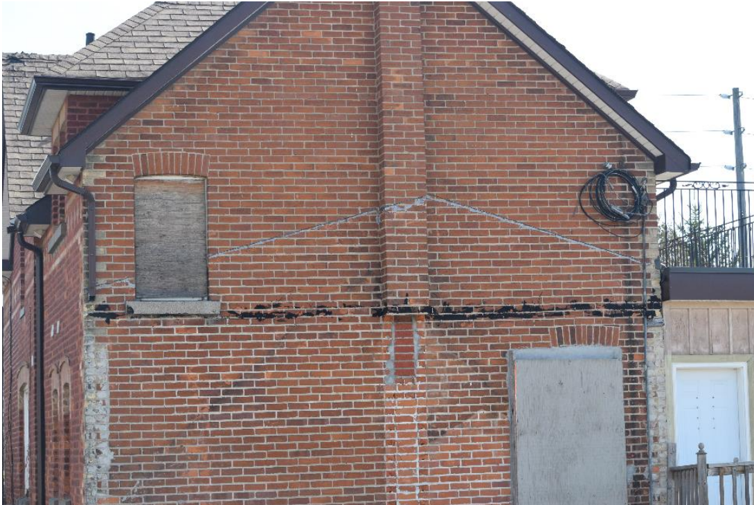
Image 25: Rear of structure showing signs of removal of previous rear addition.
