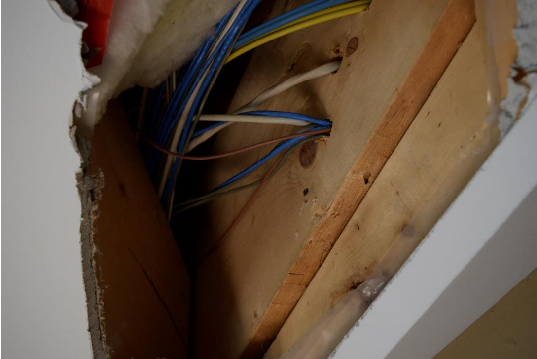
Image 47: Example of new roof framing.
