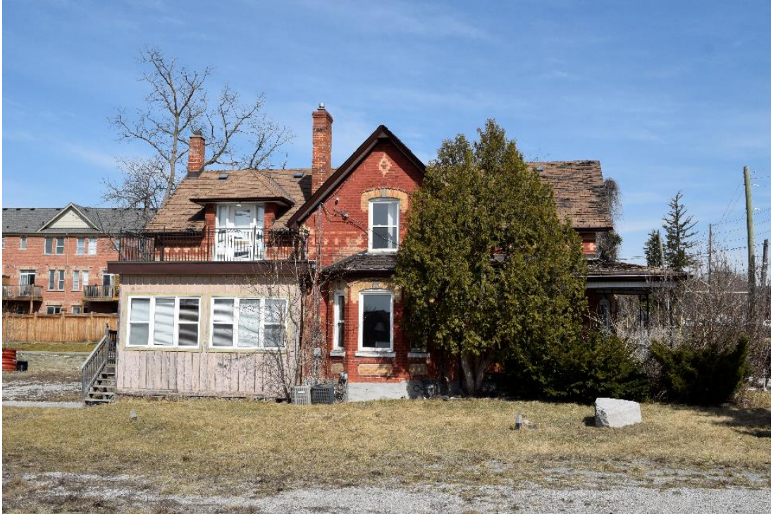
Image 10: South face of Moody-Darker House, facing north.
