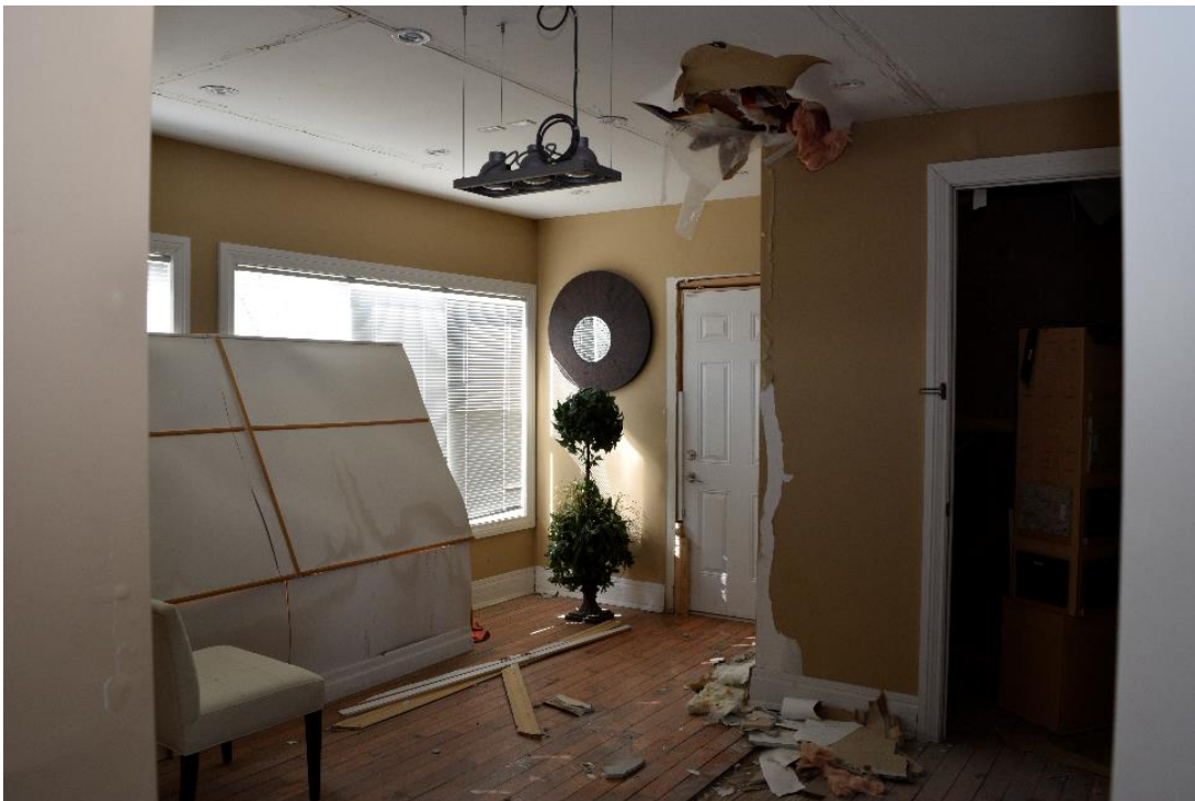
Image 40: Area where large section of wall has been removed facing southwest.
