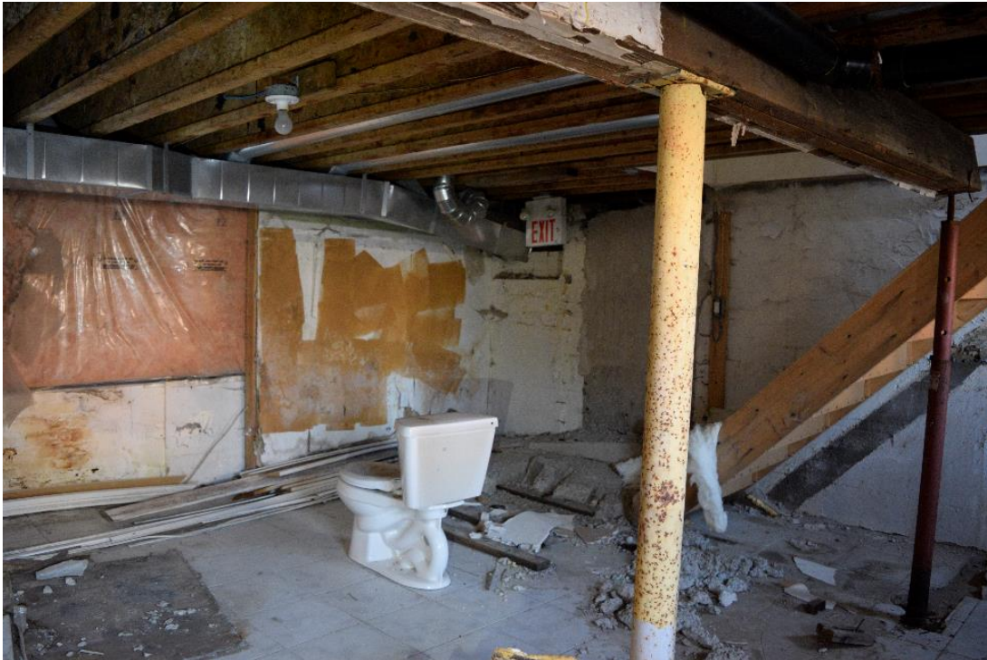
Image 51: Basement, facing southwest.
