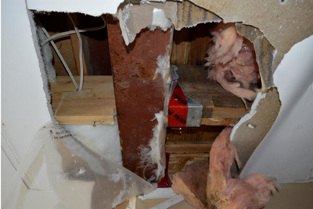
Image 41: Steel I-beam used to replace structure where wall has been removed.
