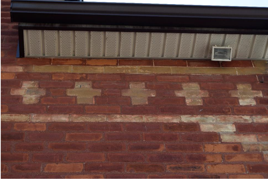
Image 19: Representative example of dichromatic decorative element on second storey.
