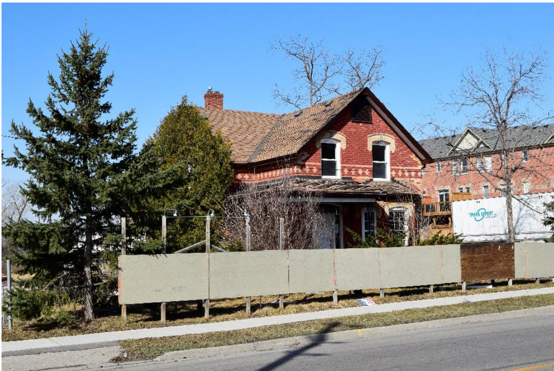
Image 11: Southeast corner of Moody-Darker House, facing northwest.
