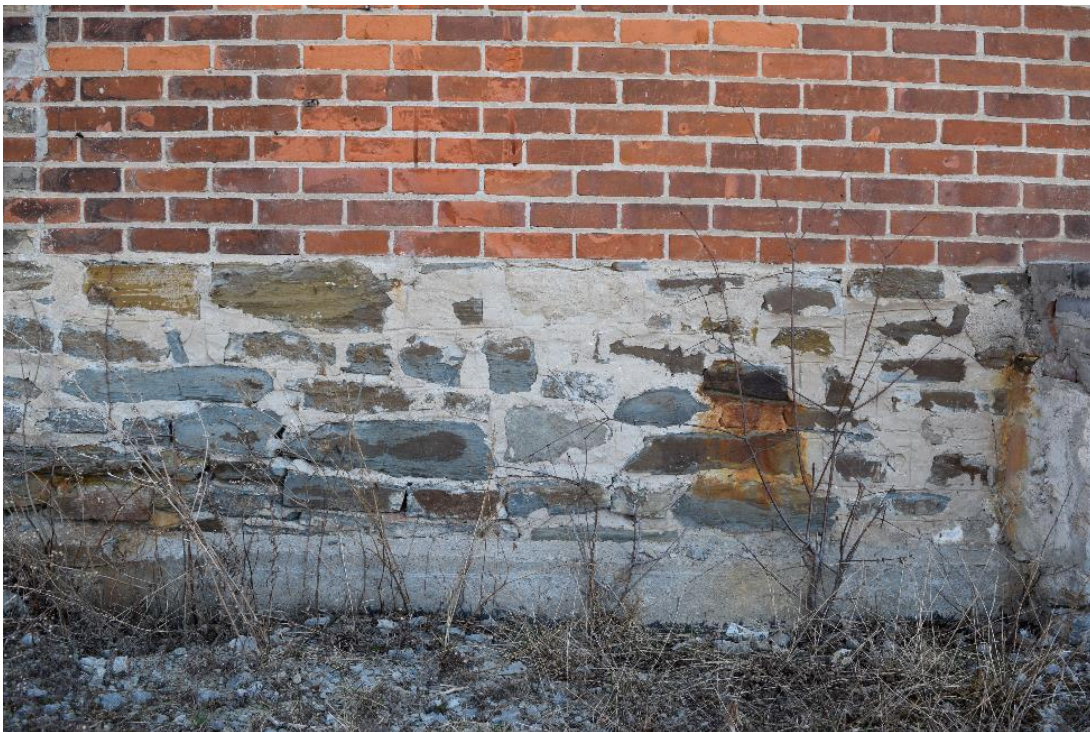
Image 24: Example of field stone foundation with flush bond mortar.
