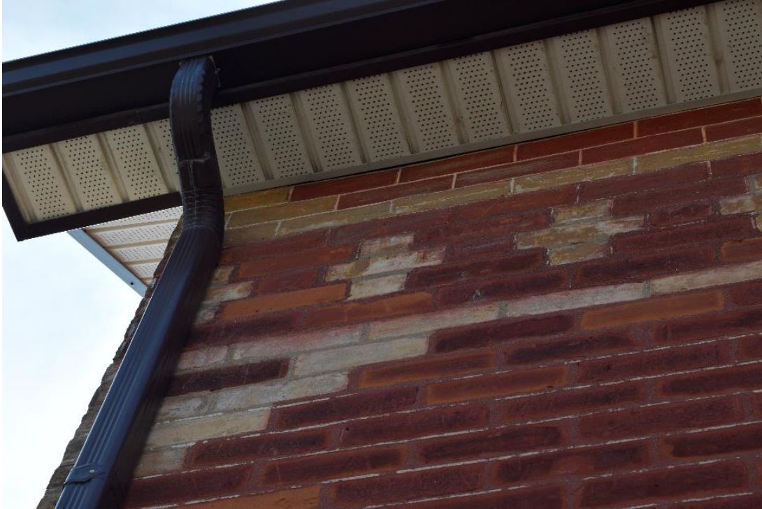
Image 23: Use of modern aluminum fascia, soffit and eavestrough.
