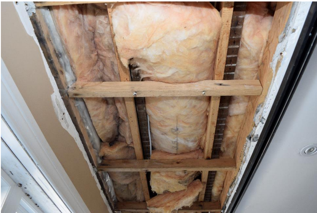
Image 37: Evidence of past renovation, note use of sistered joists.
