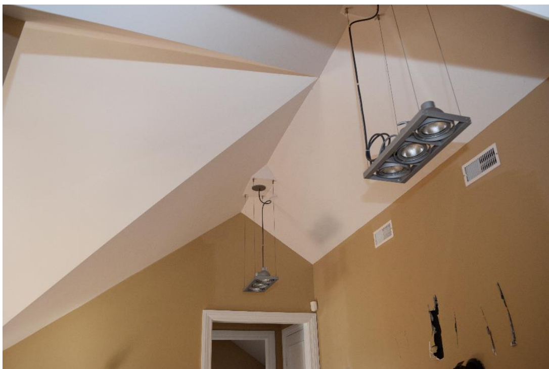
Image 44: Modern roof construction on second floor.
