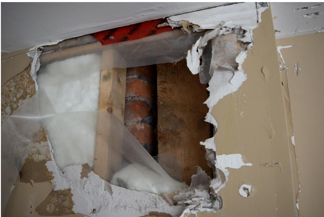
Image 48: Example of new wall framing with original brick behind.
