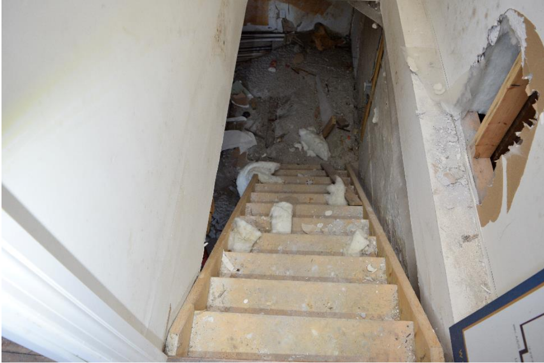
Image 49: Stairs to basement.
