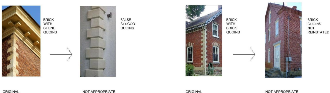
Plate 4-1: Not appropriate: Original quoins replaced with false stucco quoins or brick quoins not reinstated
