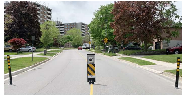
Centreline Bollards / Flex Bollards
