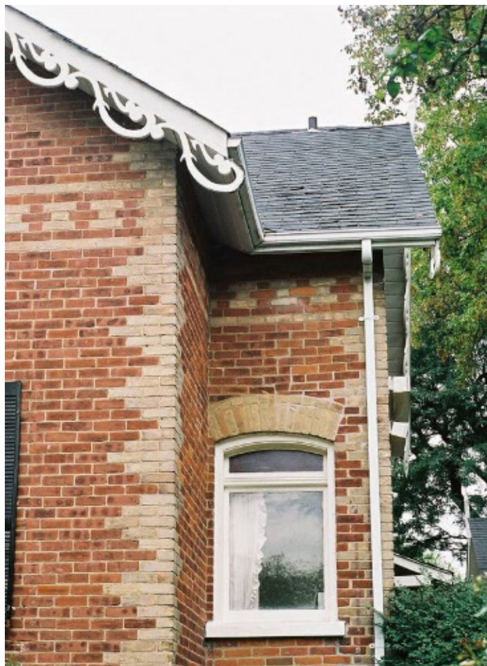
Image 45. With occasional maintenance, the wood “gingerbread” trim and windows have lasted about 130 years.
