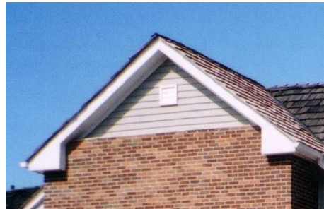
Image 26. Incorrect pre-finished metal 'box' termination
