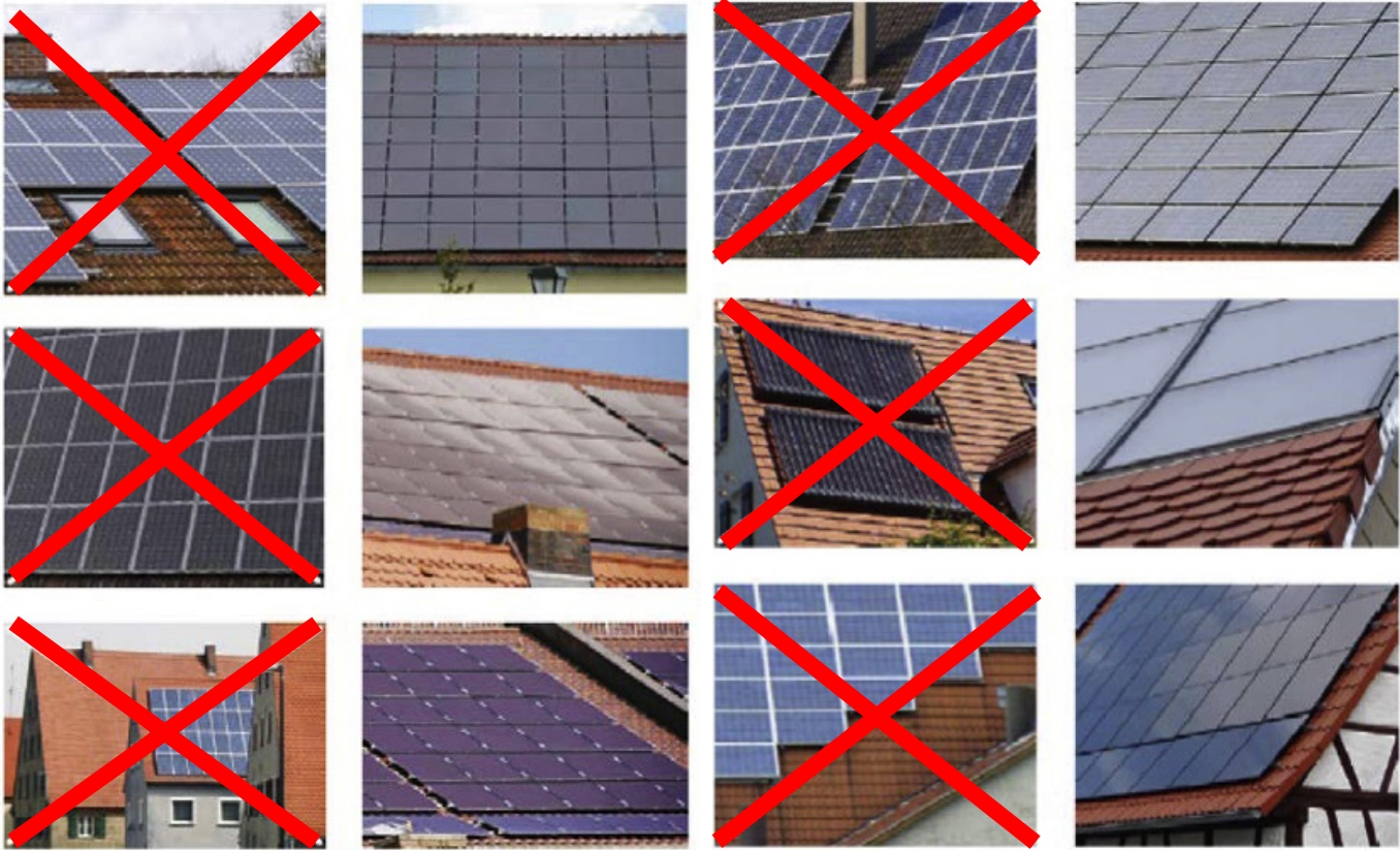
Image 63. Comparison between acceptable and not-acceptable integration of PV systems over traditional clay-based roof systems 38
