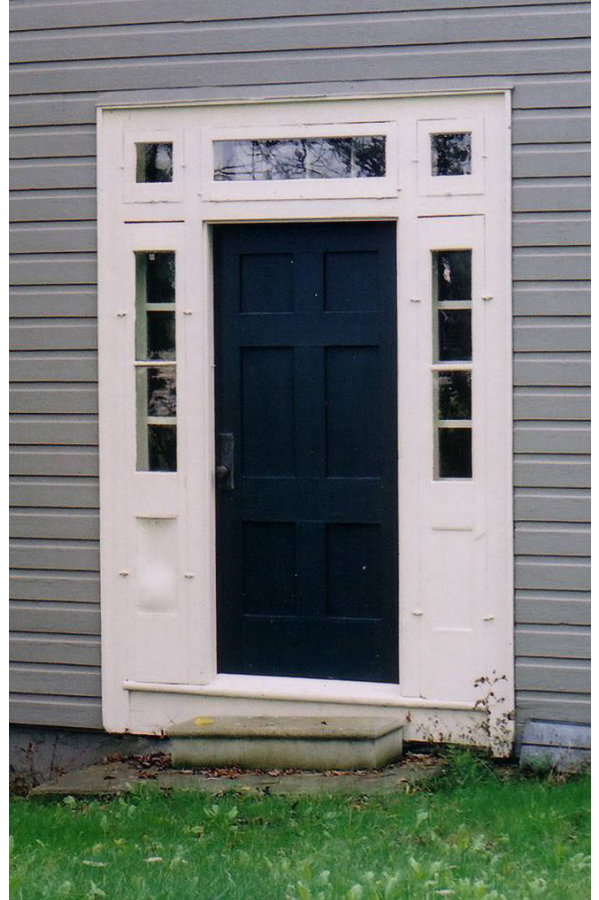
Image 46. Life-cycle costing makes wood look good. Kleinburg has many wood windows that are still in service after more than a century. This neat traditional storm window installation needs fair weather storage and occasional painting. “No maintenance” materials can’t be maintained, and need replacement when they fade, chip and dent.
