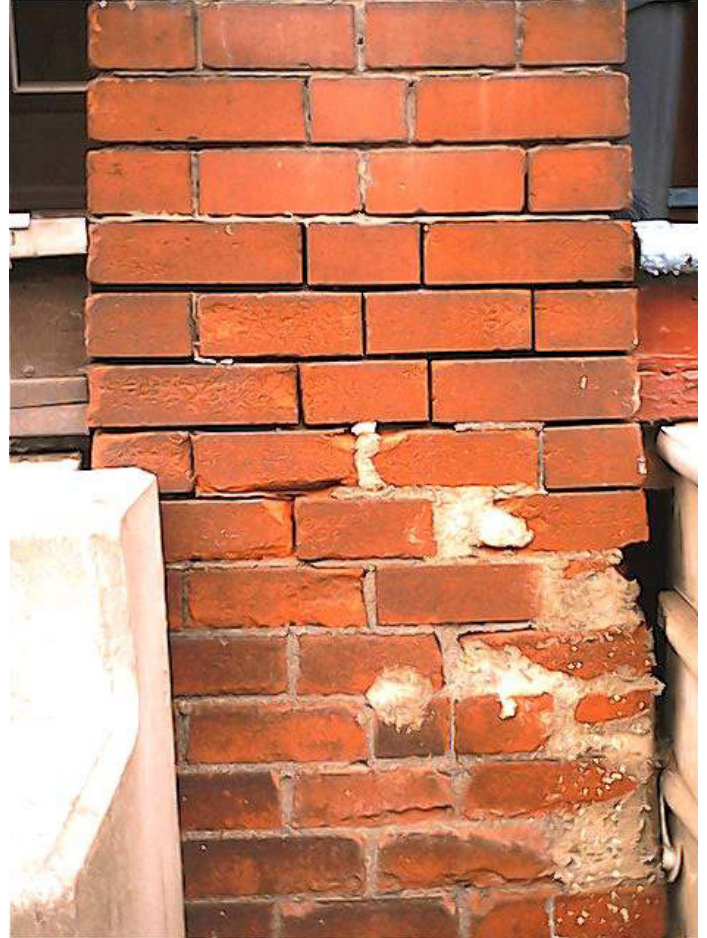
Image 44. Progressive deterioration: Rainwater splashing on the porch and steps eroded the mortar. The mortar erosion allows increasing amounts of water into the bricks and mortar below, and they are spalling and washing away, letting in even more moisture.
