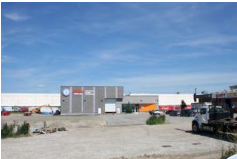
18. View from the south lot line to the north, showing the existing view from the north laneway to the south face of the tunnel training building. Surface parking will be retained between these structures.
