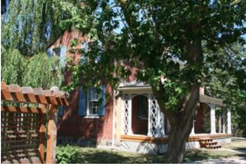
7. View of the south facade of the Robert Agar House. Tall trees situate the BHR in a mature landscaped setting. To the far left, a pergola adds to the historic character of the front (east) half of the lot.
