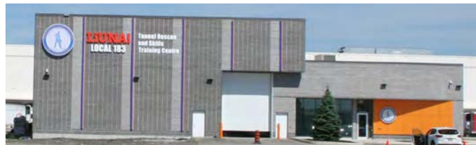
Tunnel Rescue and Skills Training Centre (ERA, August 2022).
