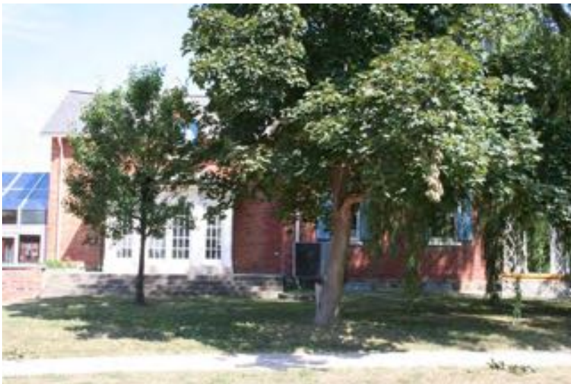
9. View of the south facade of the Robert Agar House, situated within a mature landscape setting. To the far left, the gabled glass breezeway connecting the home to the campus is visible.
