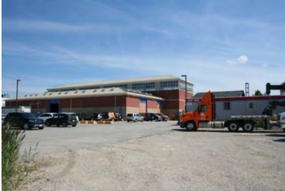
19. View of the southwest rear campus extension. The proposed storage building would be situated roughly where the transport trucks are pictured in this image.
