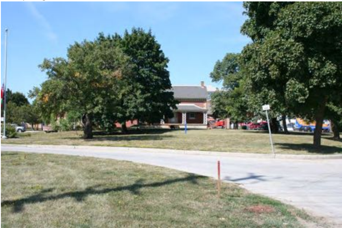
4. View of the east facade of the Robert Agar House. Note the mature vegetation that situates the BHR in a picturesque context while obscuring views of the contemporary LiUnaA campus behind.
