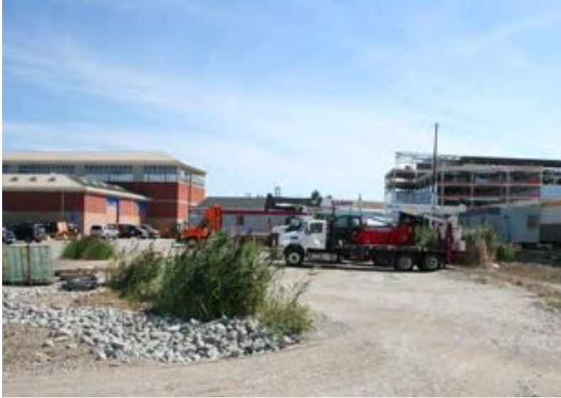
16. View of of the rear campus extension from the southwest curve of the laneway. The proposed storage building would be situated near the visible transport trucks in this image.
