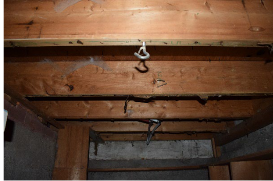
Plate 40: Basement planed dimensional lumber floor joists
