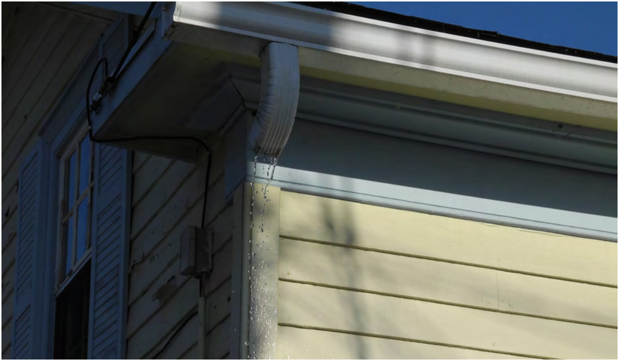
Figure 16: Eaves and disconnected downspout at south-west corner of Main House, showing water discharging directly onto the cladding (CBCollective, 2020).
