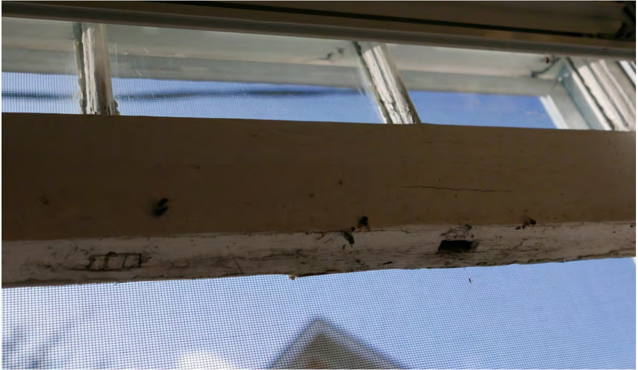
Figure 22: Detail of the bottom rail on the west elevation's south window. The muntin bar's wedge-tenon has broken off and is missing. Sash is still structurally sound but should be repaired ( CBCollective, 2020 ).
