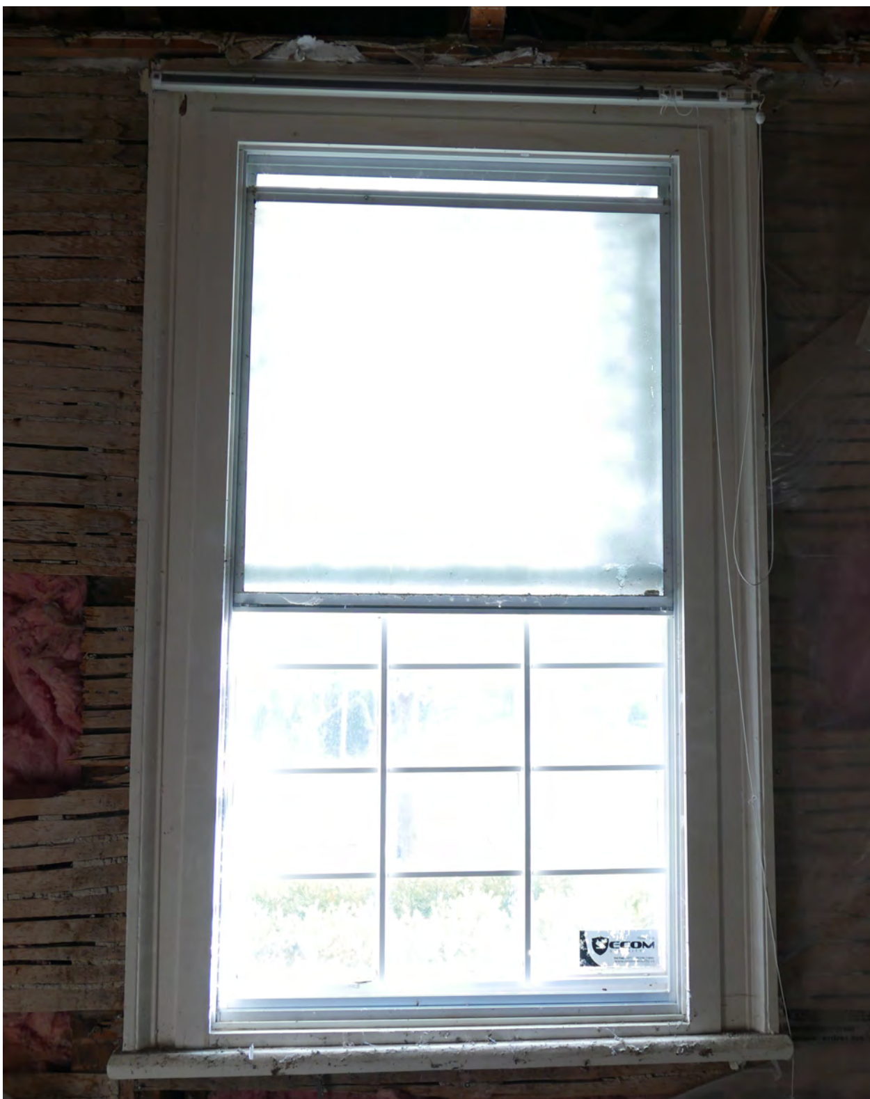
Figure 26: Historic casings remain at the Main House's interior windows, despite being obscured by storm windows. Profiles differ slightly on the ground floor windows (CBCollective, 2020).
