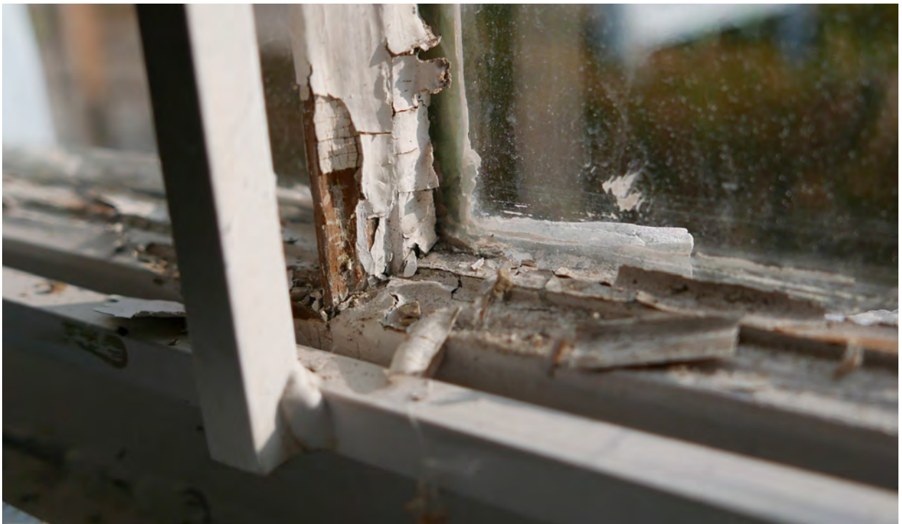
Figure 21: Detail of south-east window, showing paint failure where the muntin bar is mortised into the rail. The wood is in good condition at this location, and older crazed finishes are visible ( CBCollective, 2020 ).
