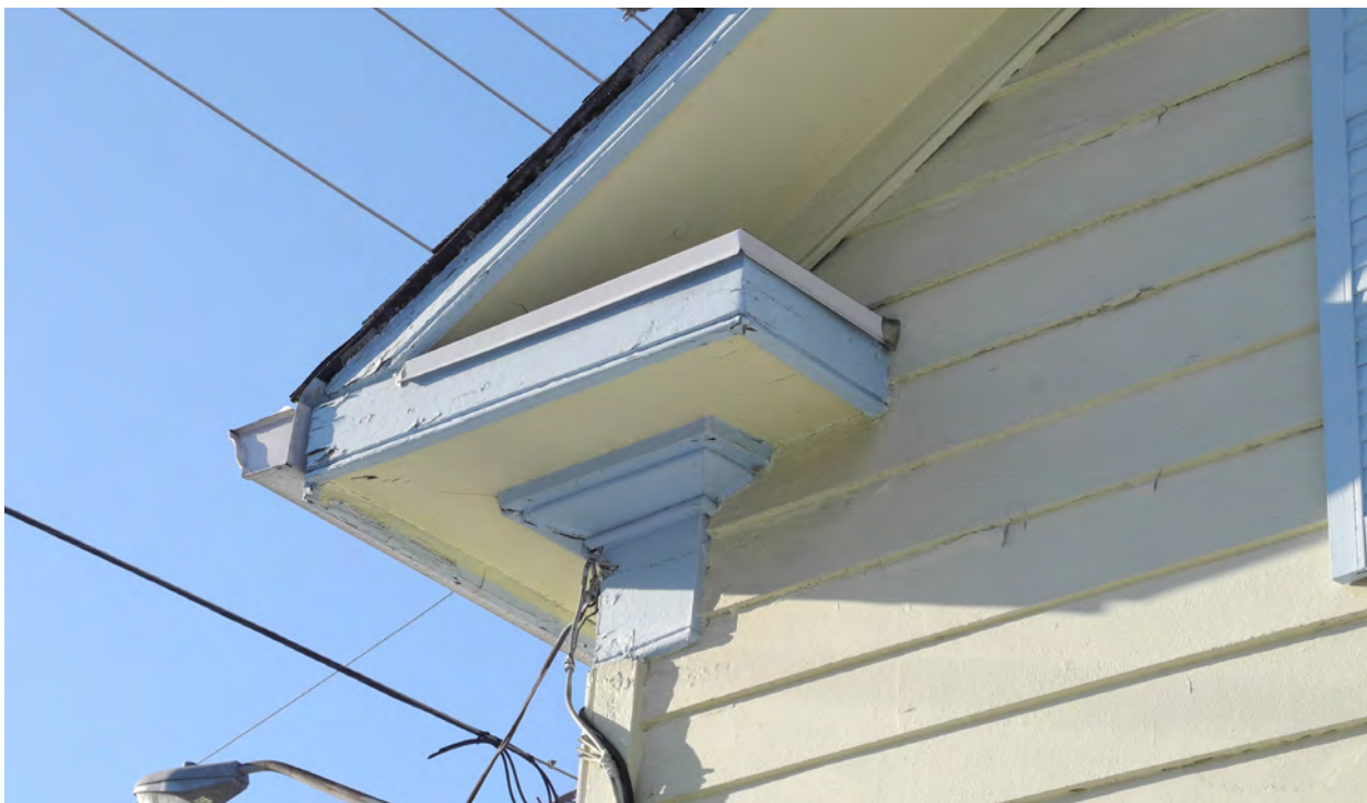
Figure 18: Detail of fascia and soffit at south-east gable return. Soffit boards are in good shape overall and display paint failure. Oversized fascia boards are apparent on the south elevation (CBCollective, 2020).
