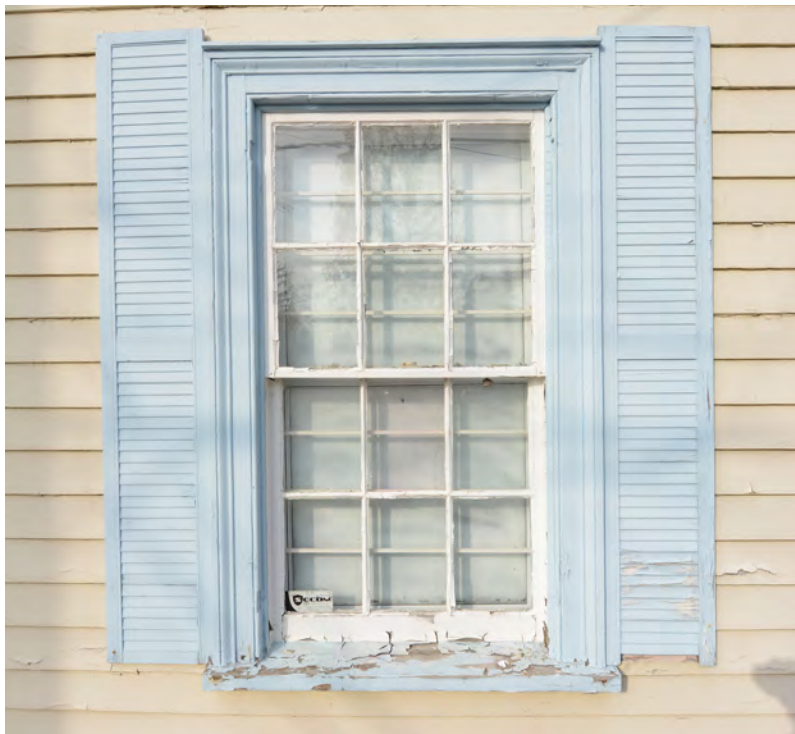
Figure 8: East window on the Main House's north elevation, showing typical configuration, casings, sill and shutters. Hinge mortises from earlier functional shutters can be seen on the inside of the left casing (Michael Scott Architect, 2020).
