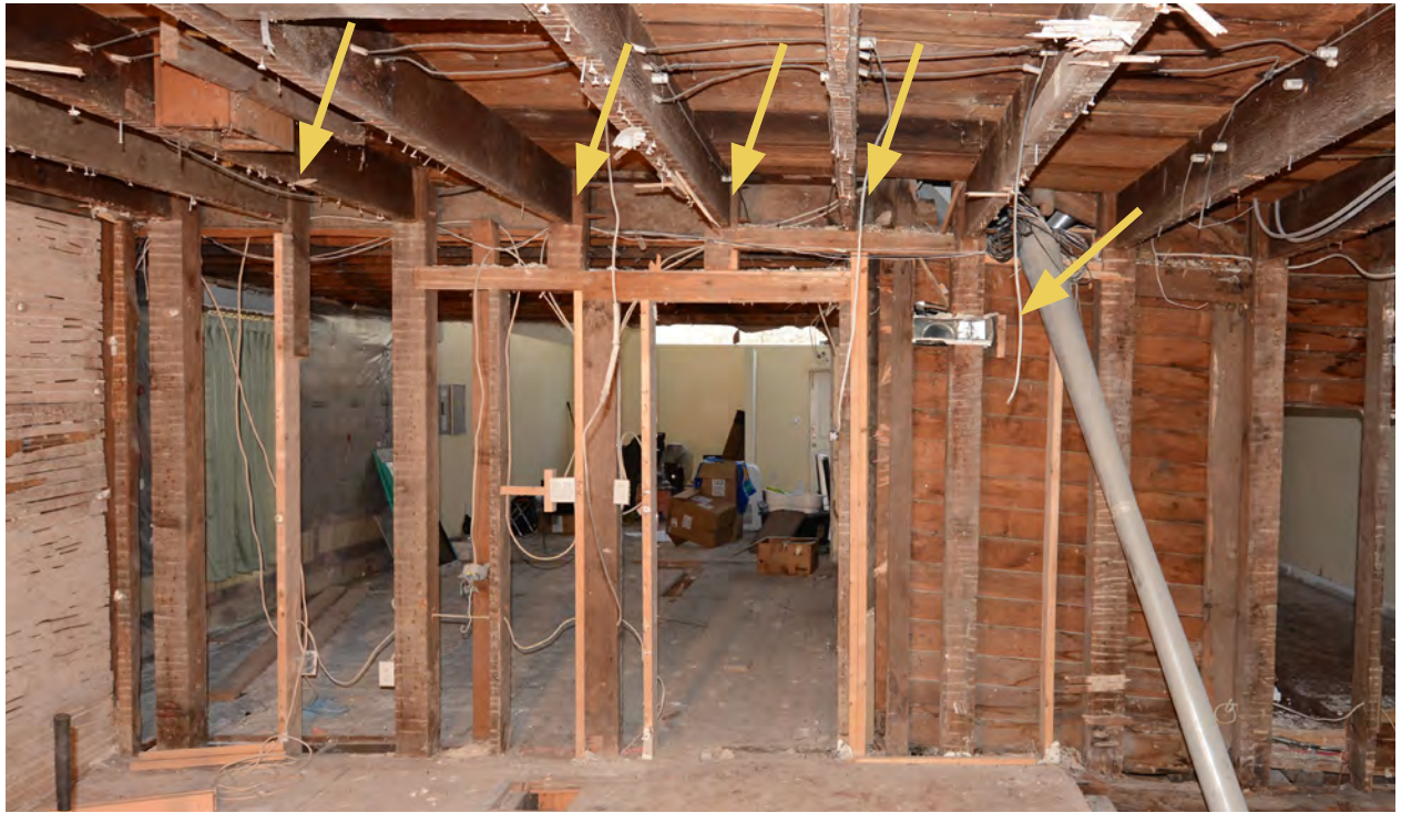
Figure 12: Photograph of Main House's north wall showing numerous and significant modifications to the original framing system. Yellow arrows indicate original posts that have been modified or severed ( Michael Scott Architect, 2020 ).
