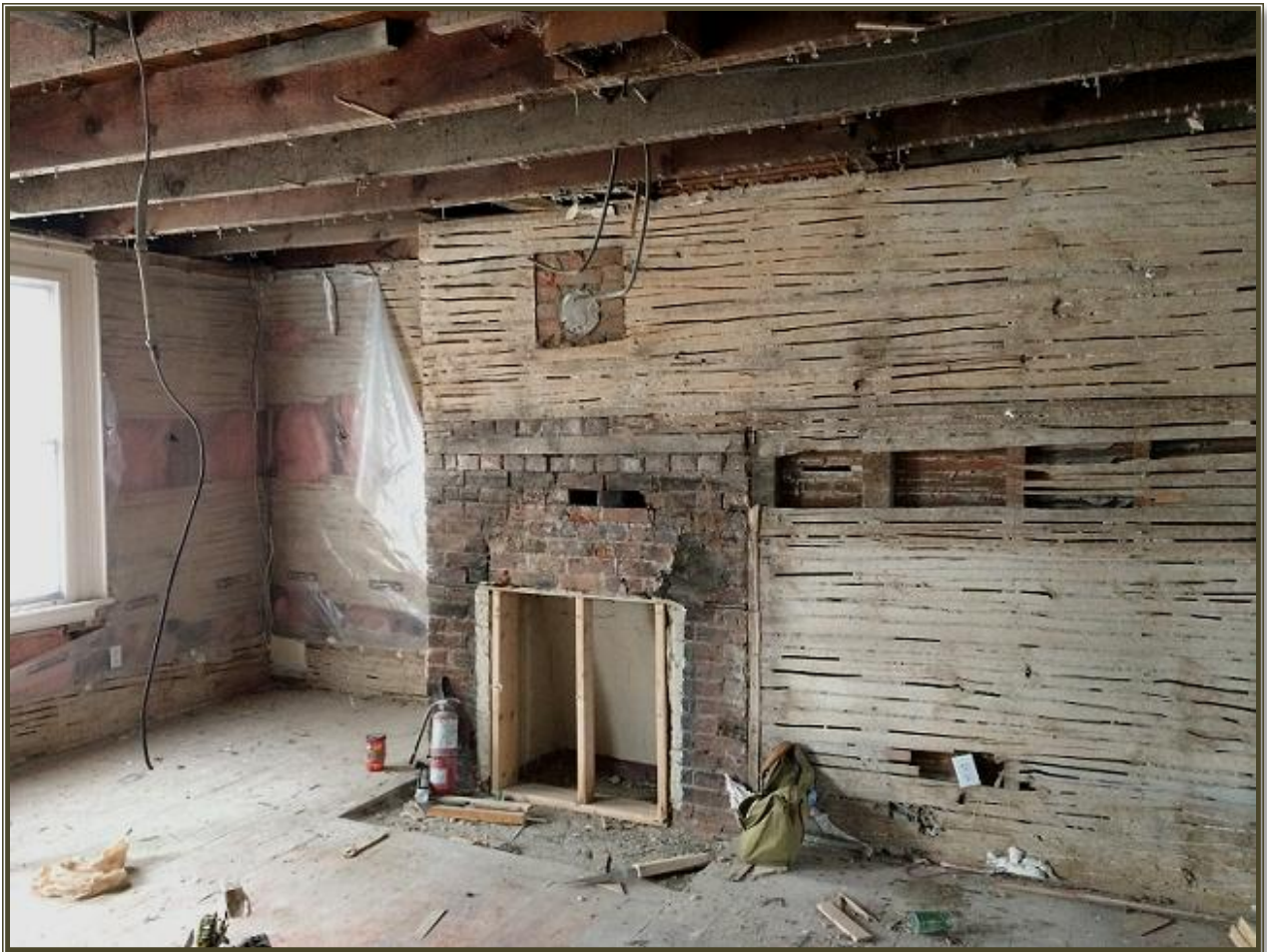
5.4.4 Brick fireplace opening, 4" x 4" and 2" x 4" framing, split lath, 15 November 2017. This is a character-defining attribute of the subject property. Void behind lathed wall is stairway to upper floor per Figure 5.4.8, below.
