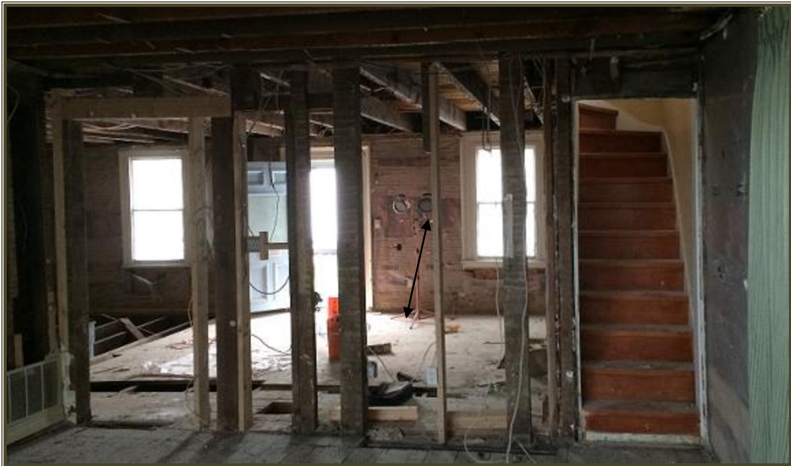
5.4.8 Looking south from tail addition toward front wall of house through various thicknesses of framing, 15 November 2017. Note winding stair at right and lath markings on addition side of framing.
