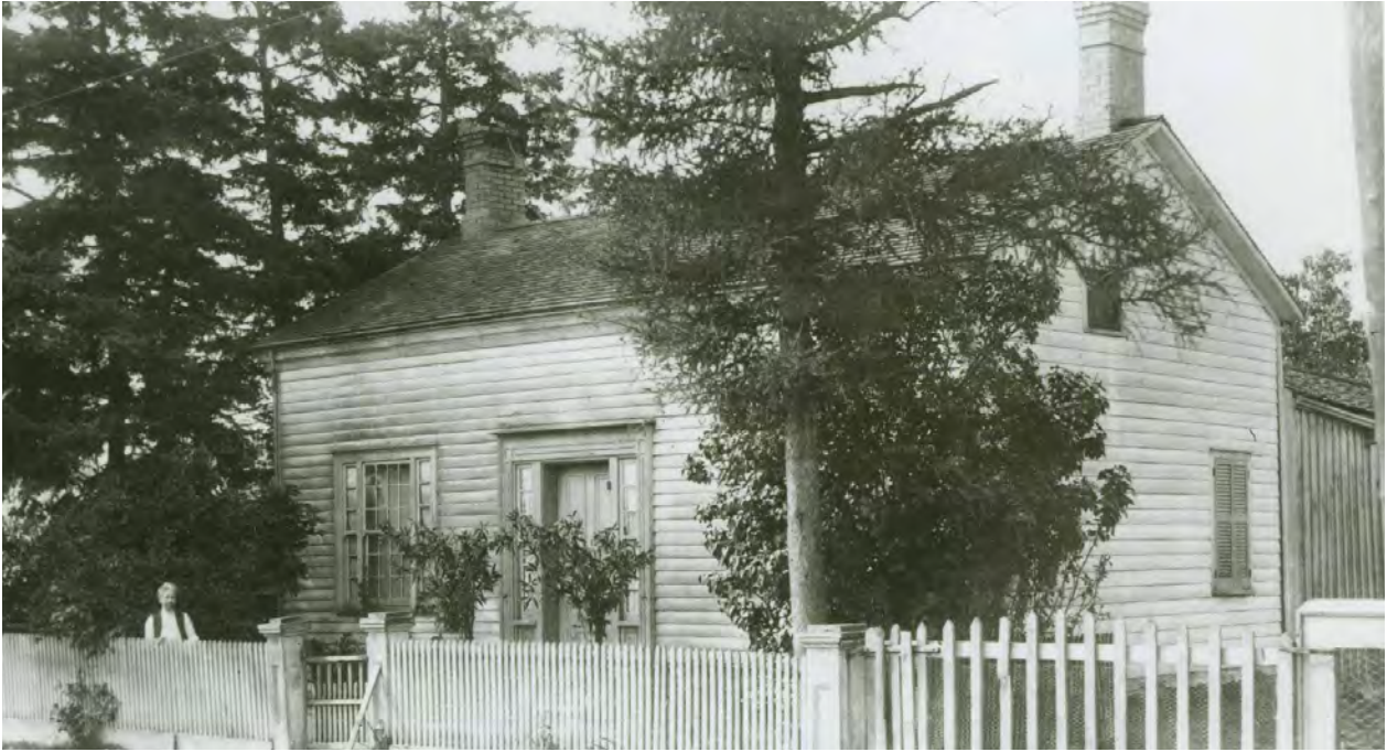
Figure 3: William Watson house, c1900. The vertical board and batten siding of the addition differentiates it from the main house which is clad in horizontal wood siding. Source: Thornhill Archives, Weaver Collection, Thornhill Houses and Buildings.
