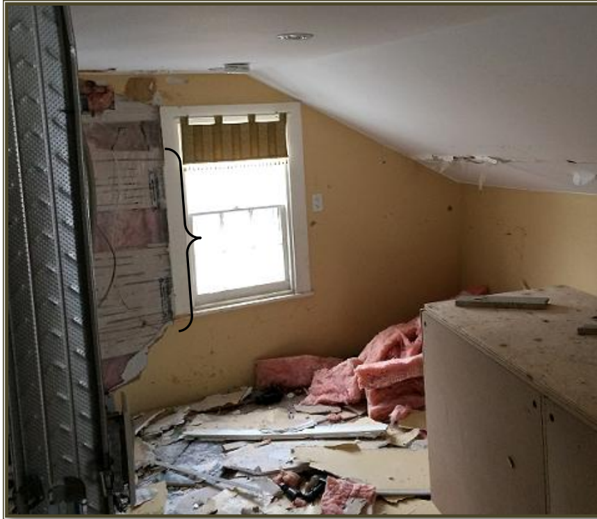
5.4.21 South window of upper half-storey of probable original mass with wood lath (bracketed), 15 November 2017.
