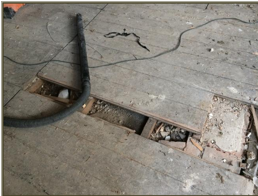
5.4.10 Per red dashed line above, view of relationship between floor joists and soil, 15 November 2017.
