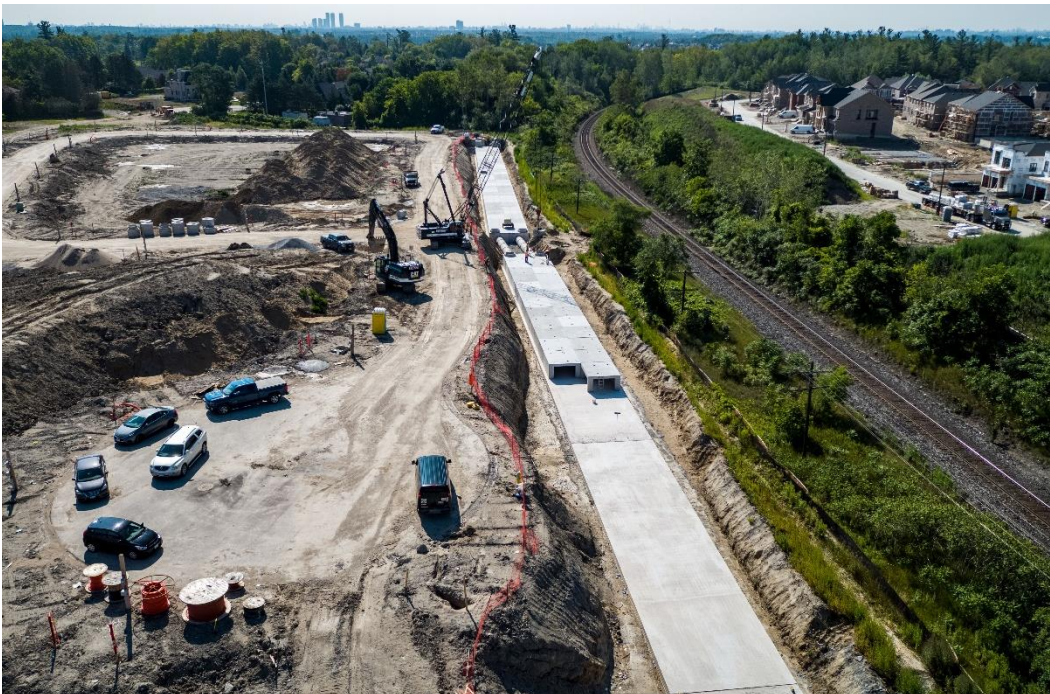
Source: DECAST, Installation of UG/SWMF in the City of Vaughan
