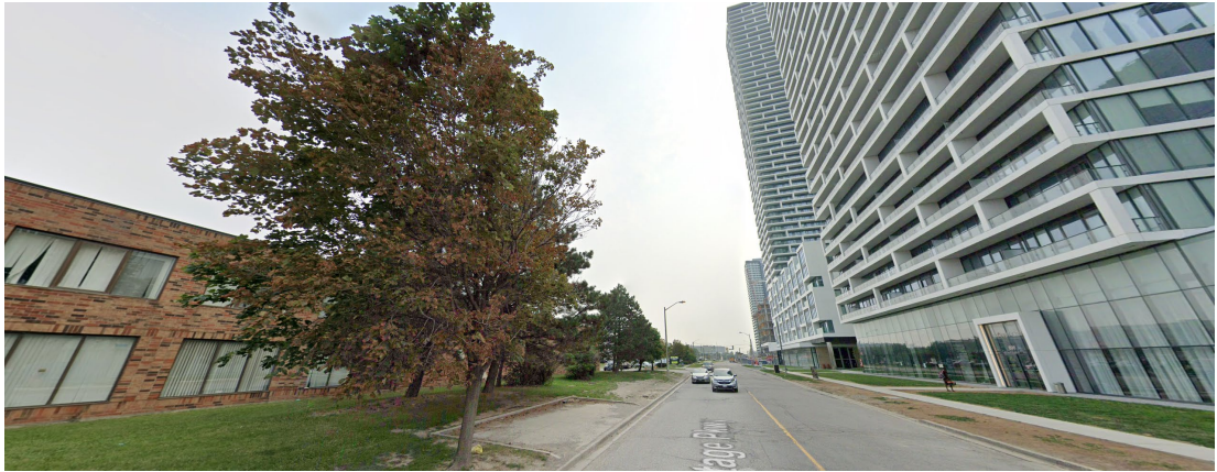
Image 2/ View of Portage Pkwy looking east just before Millway Avenue
