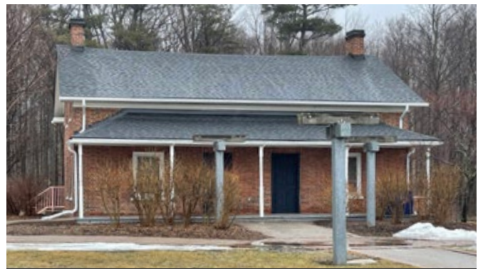
Baker Homestead roof replacement
