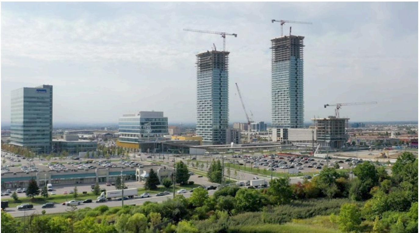
Vaughan Metropolitan Centre construction
