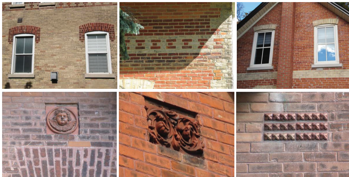
Photo 4-3: Examples in Core Maple HCD of red and buff brickwork and brick detailing including voussoirs, drip moulds, horizontal banding, quoins, and decorative clay elements in brickwork
