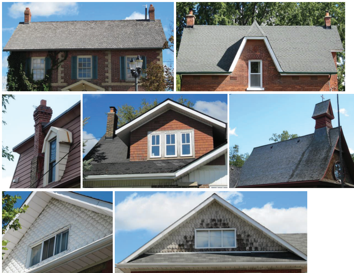
Photo 4-1: Examples of roof materials, shapes, pitches, and other elements in the HCD (chimneys, dormers, cupola)
