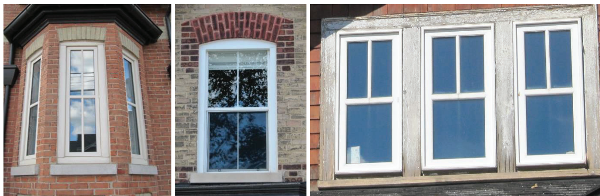
Photo 4-7: Examples of appropriate replacement windows in HCD including fixed sash, 2/2 sash windows within a segmental frame, and 2/1 fixed windows within original wood frames
