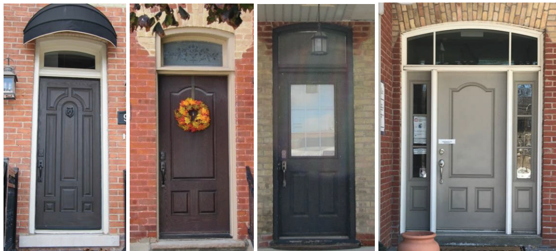
Photo 4-9: Examples of appropriate replacement doors in the HCD that retain the original door shape, transom, sill, and voussoir details
