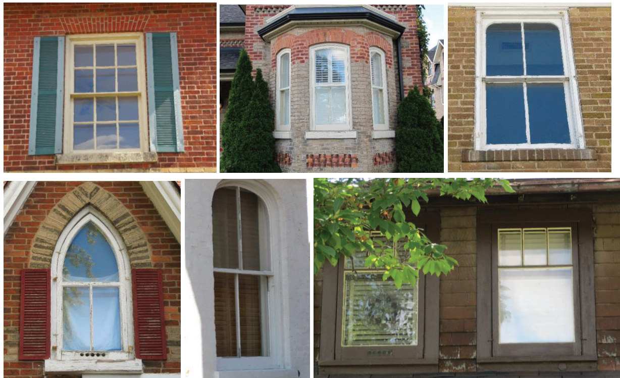
Photo 4-6: Original window examples in HCD including rectangular multi-sash, segmental storm windows, semi-elliptical sash, pointed arched, semi-circular sash, and rectangular 3/1
