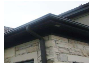
SOFFIT, FASCIA, DOWNSPOUT
