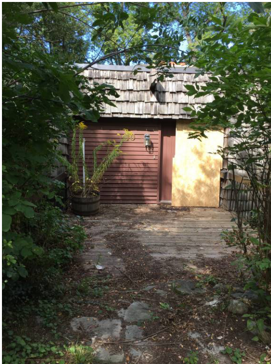
Figure 11. Front entry. Plywood covers broken sidelight. Due to dense vegetation, this is about all that is visible from the roadway.
