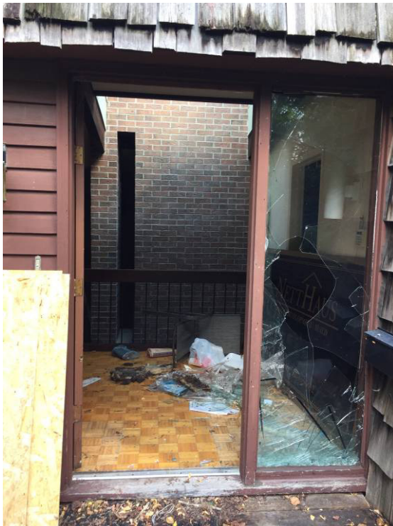
Figure 12. Plywood removed, showing broken glass.
