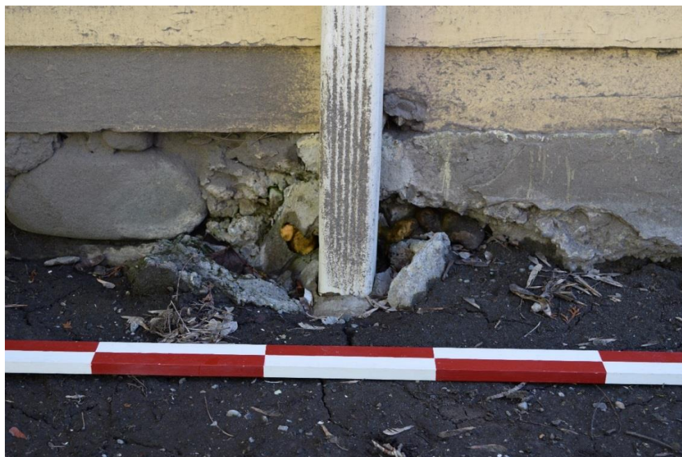
Figure 46: Mortar and concrete damage on the north foundation wall at a downspout location.
