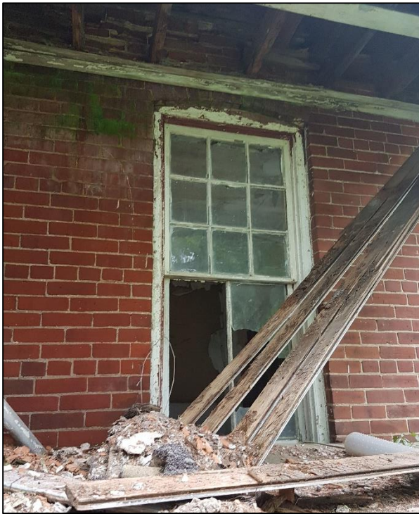
Figure 40: East elevation detail showing the window opening beneath the porch roof and open rafters above
