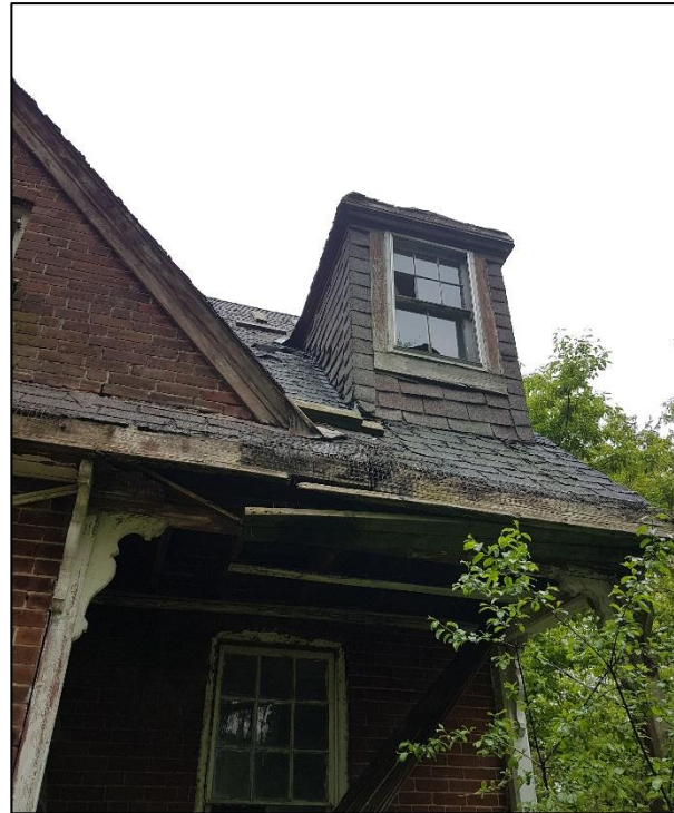
Figure 41: East elevation detail showing the deteriorated porch roof and dormer above the porch
