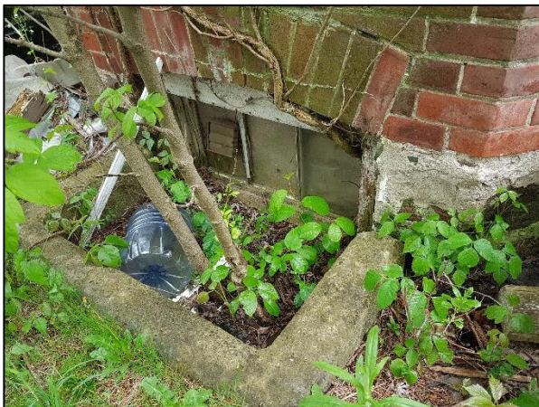
Figure 34: East elevation detail showing segmentally arched basement window openings and parged foundation (ASI 2019)
