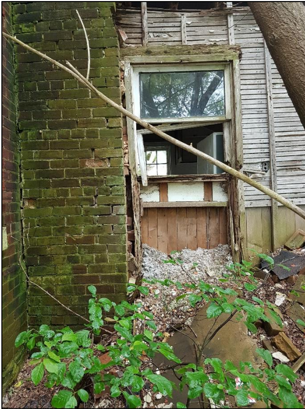
Figure 46: North elevation detail showing deteriorated exterior wall and first-floor window opening (ASI 2019)
