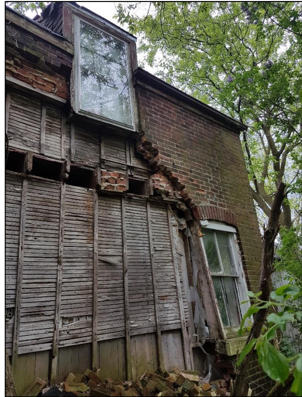
Figure 47: North elevation detail showing deteriorated and missing exterior wall, dormer window and first-floor window opening (ASI 2019)
