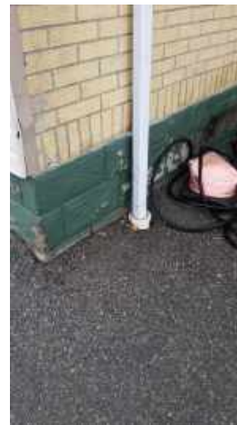
Downspout below grade discharge
