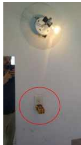
Inoperative outlet (also exposed bulb above)
