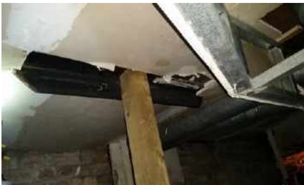
Steel angle-iron installed under floor joist and propped up by wood post
