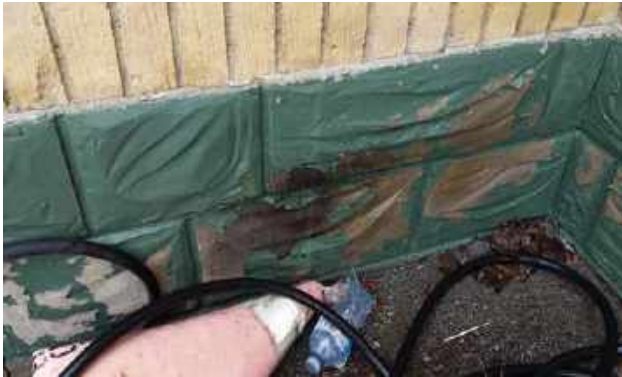
Concrete block above grade. Note surface mold on saturated block.
