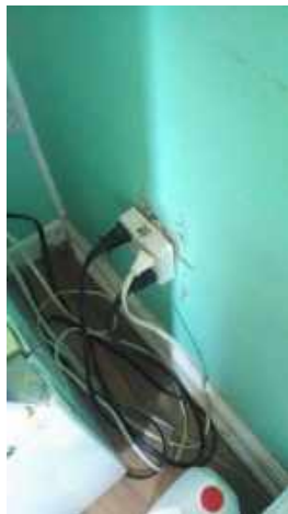
Wall outlet likely overloaded
