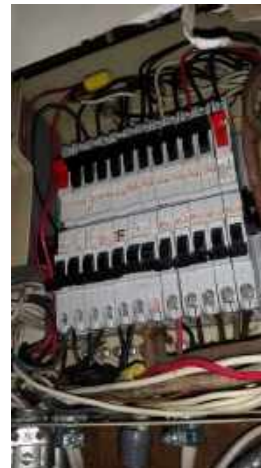
Panel noted as full. No spare circuits / breakers available
