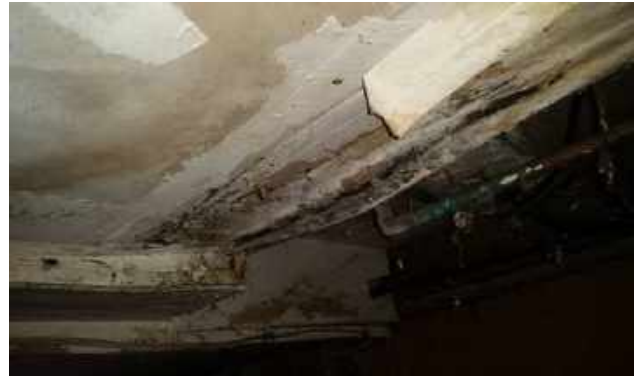
Drywall on basement ceiling is damaged by moisture. Mould growth also visible.
