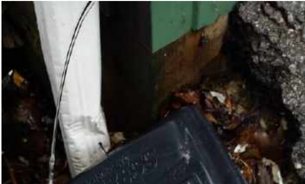
Wood to soil contact in north east corner of building
