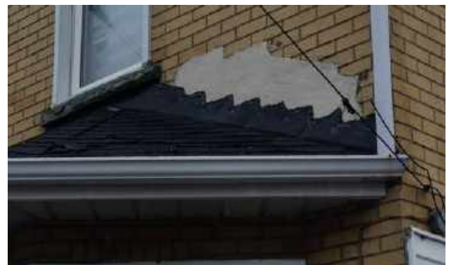
Parged wall above flashing
