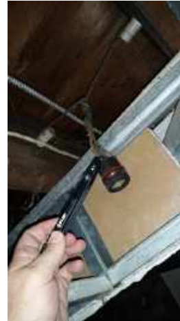
Old active knob and tube wiring
