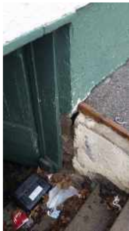
Damaged foundation wall at basement walk-out
