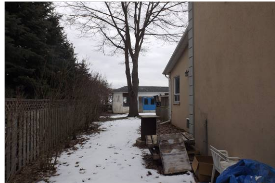
Figure 12. View from the north. Ad-hoc frame rear vestibule. Original brick on the right, and at ground floor on the left. Window opening not original.
