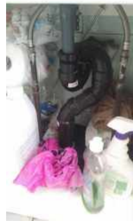
S-Trap drain configuration under main floor bathroom sink
