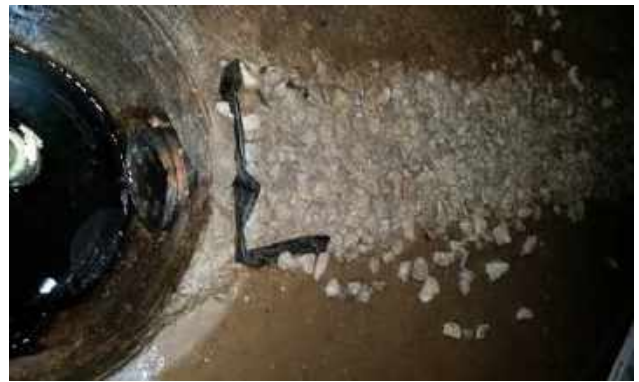
Trench / drain pipe leading into sump pit
