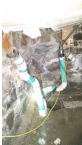
Cast iron and brass connection to newer PVC type drain pipe in basement
