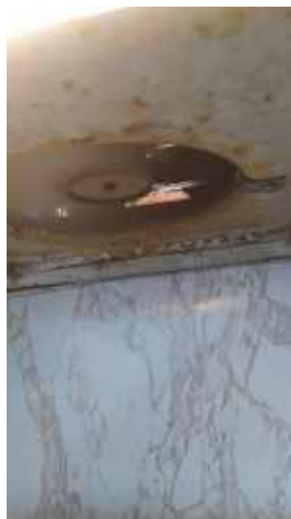
Rusty old fan above stove with no filter elements and direct view to exterior.
