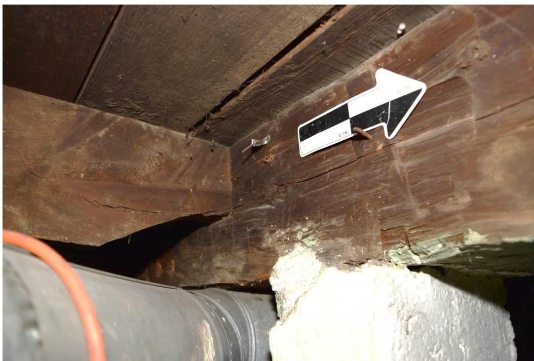
Figure 35: Notching of the Main Block sill to accommodate a floor joist.
