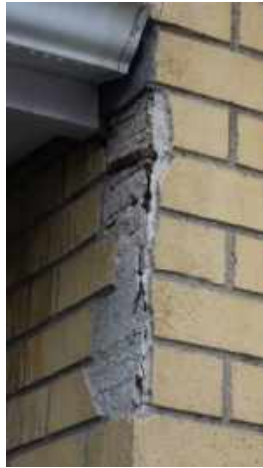
Missing area of brick tile exposing cement substrate and mesh
