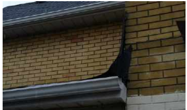
Improper wall flashing
