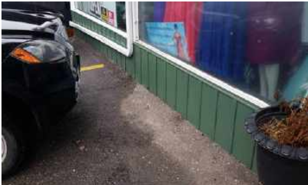
Paving installed against siding
