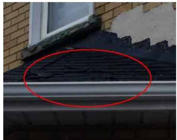
Some shingles deterioration noted in places. Likely due to moisture penetration.
