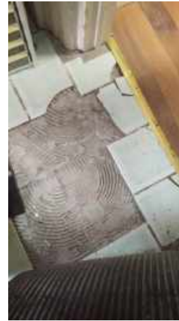
Cracked / broken floor tile
