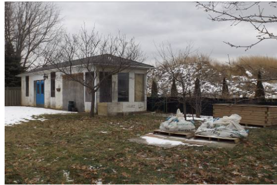
Figure 11. View from west. Original brick, but no original window openings.
