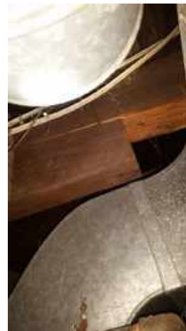
Cracked / compromised floor joist
