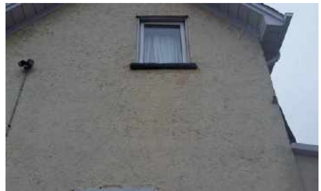
Rear stucco wall. Discoloration, especially under window sills noted.
