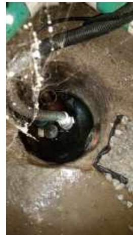
Pump discharge tube runs into foundation
