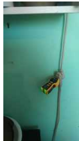
Extension cords used as permanent wiring
