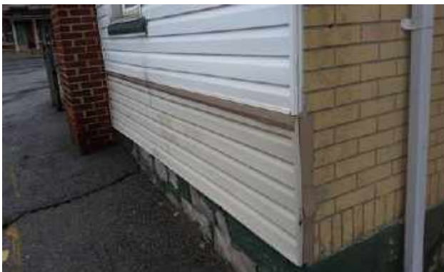
Siding type over brick tile varies as applied at different times.
