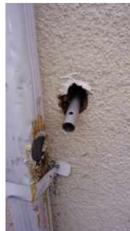
Damaged / perforated downspout
