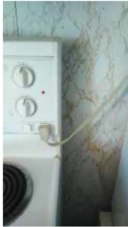
Stove outlet also used for small appliance
