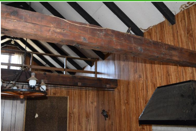
North main room with exposed squared log tie beams
