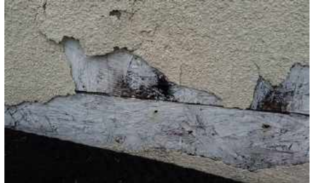
Peeling stucco due to moisture. Visible mold growth on surface of OSB.
