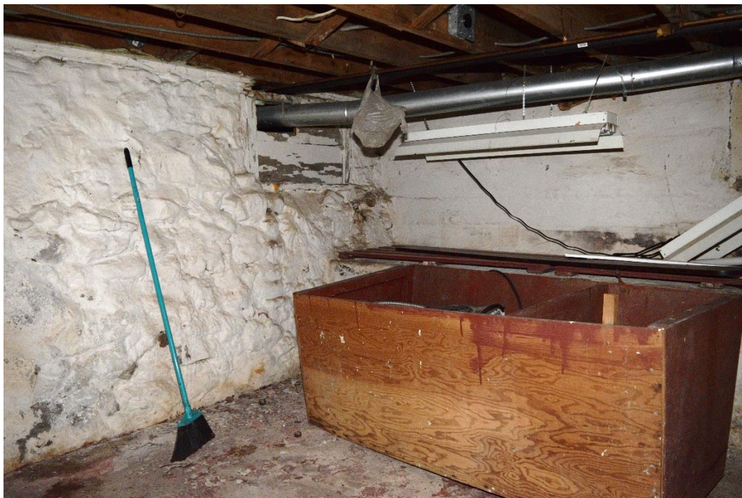
Figure 33: The rounded fieldstone foundation as seen from beneath the West Wing Extension.
