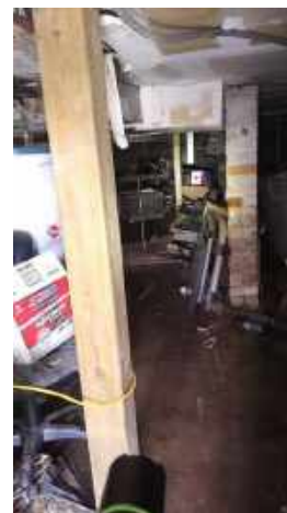
Vertical wood post supports noted in basement
