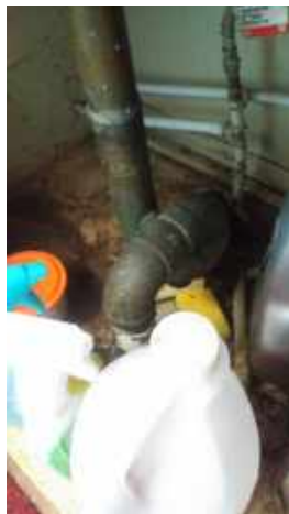
S-Trap drain configuration under main kitchen bathroom sink
