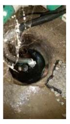
Pump discharge tube runs into foundation
