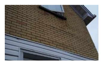
Wall area below window sill failing. Brick tile finish is buckling.
