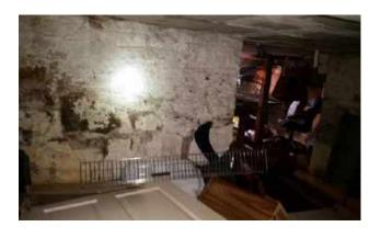
Water stained / damaged foundation wall
