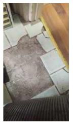
Cracked / broken floor tile
