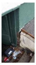
Damaged foundation wall at basement walk-out
