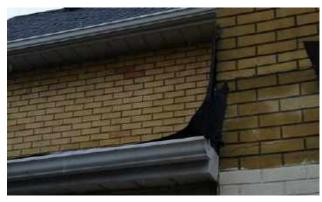
Improper wall flashing at lower roof plane
