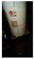
Electric HWT on concrete blocks in basement
