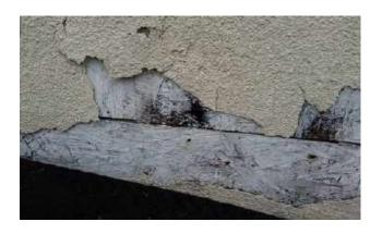
Peeling stucco due to moisture. Visible mold growth on surface of OSB.
