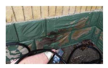
Concrete block above grade. Note surface mold on saturated block.
