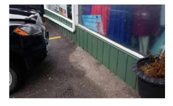
Paving installed against siding
