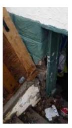
Cracked / broken foundation wall at basement walk-out
