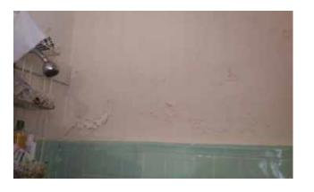
Wall above shower stall with deteriorated plaster / peeling paint
