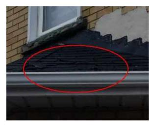
Some shingles deterioration noted in places. Likely due to moisture penetration.
