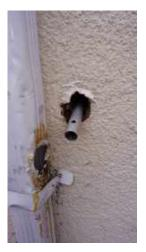
Damaged / perforated downspout
