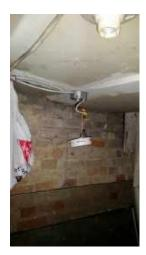
Smoke detector in basement hanging from junction box
