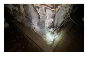
Significant amount of efflorescence on inside of foundation wall caused by moisture migration through the wall
