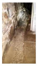
Perimeter trenching along inside of foundation wall
