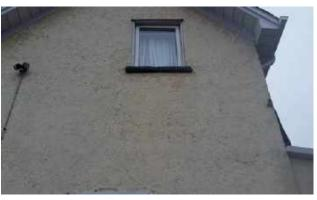
Rear stucco wall. Discoloration, especially under window sills noted.
