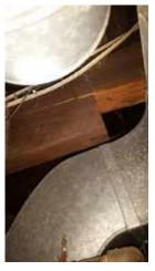
Cracked / compromised floor joist
