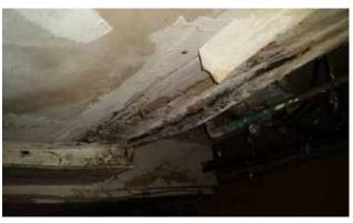
Drywall on basement ceiling is damaged by moisture. Mould growth also visible.
