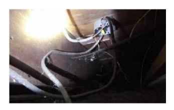
Old wires spliced with new in open junction box
