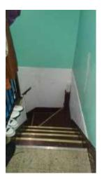
Section of stairs with missing handrail
