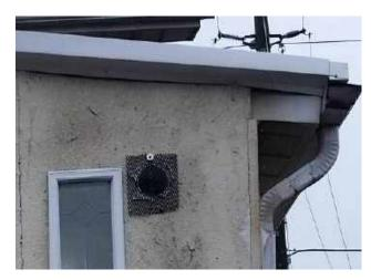
Exterior unprotected dryer vent
