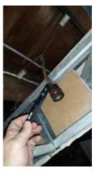
Old active knob and tube wiring
