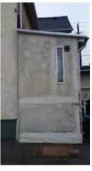
Rear wall of porch enclosure. Dark areas indicate water penetration into substrate material.
