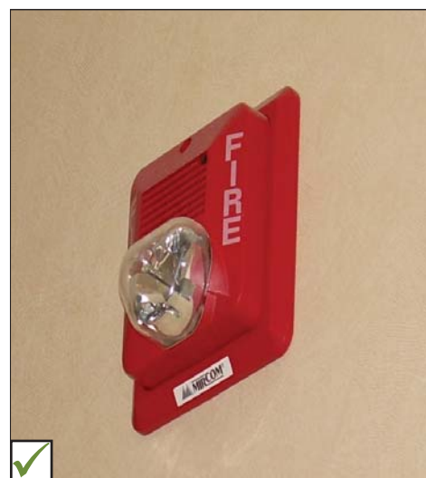
Example of combined visual and audible alarm signals. Public facilities should have both visual and audible fire alarm systems strategically located.
