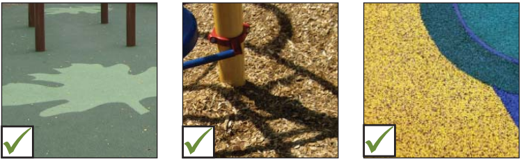
Examples of inclusive play space ground surfaces. From left to right: poured-in-place rubber, engineered wood fibre and shredded rubber.
