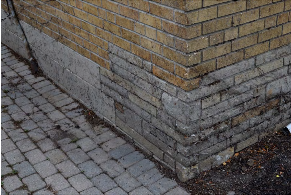
Image 11: Cement block foundation of north addition with decorative ashlar cement block used on front facade
