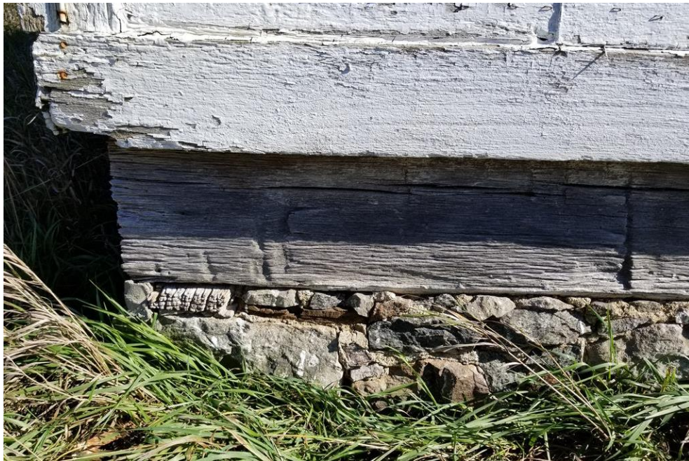
Figure 21: Coursed rubble foundation of the Main Block.
