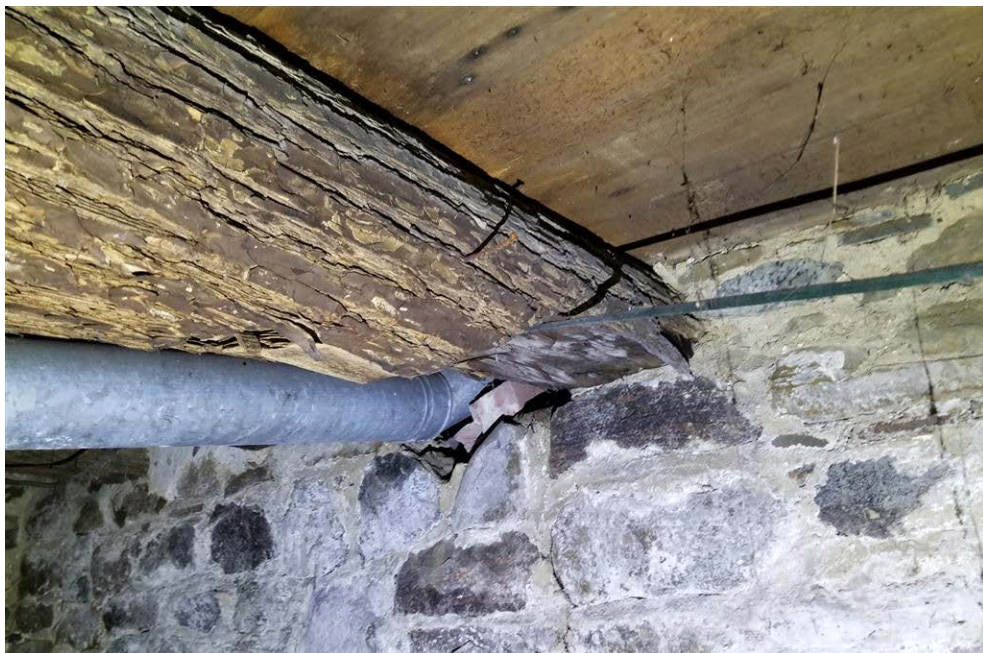
Figure 16: Example of overhead sleeper.
