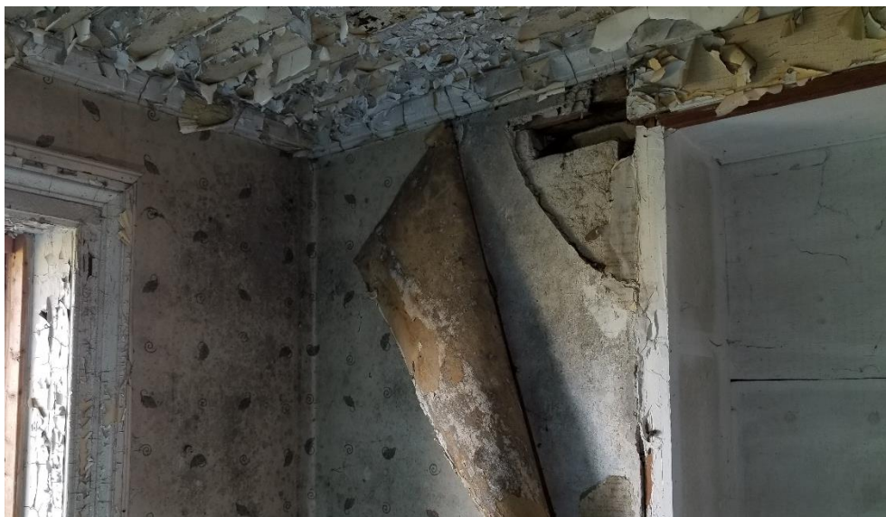
Figure 52: Bricks visible behind wallpaper and plaster, southeast corner of the ground floor room.
