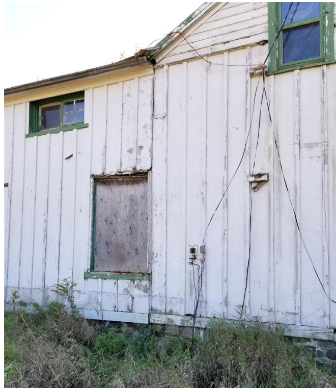
Figure 48: Visible join between East Wing and Main Block. Note the small horizontal sliding window.
