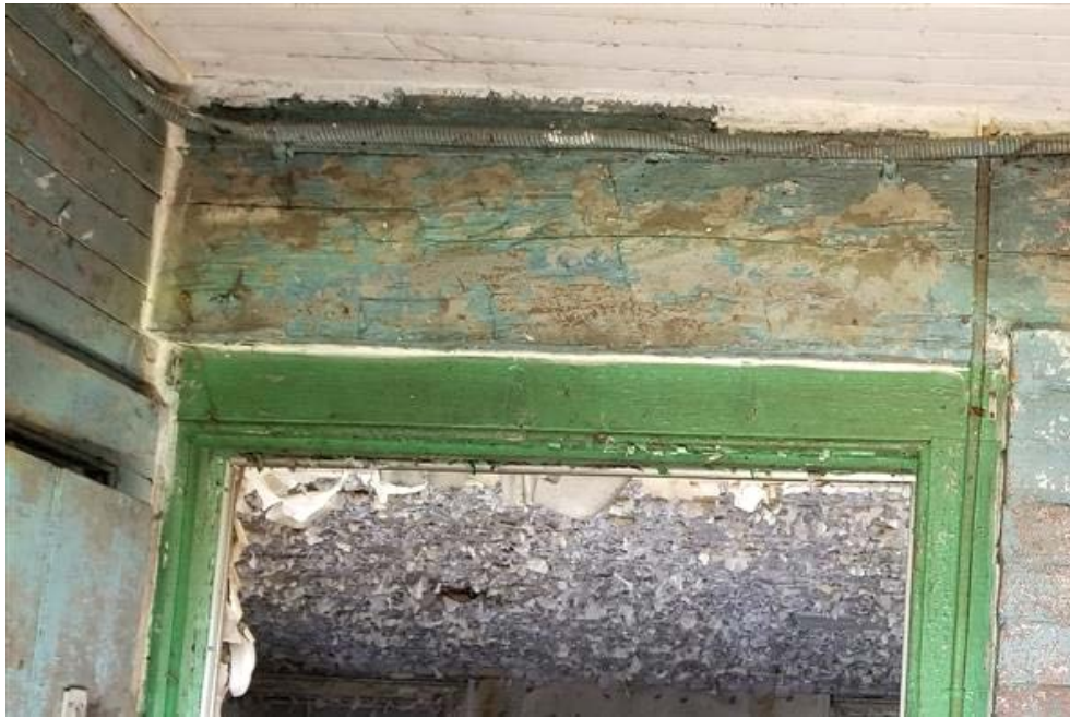
Figure 30: Adze marks on wood lintel above the door to the South Addition.
