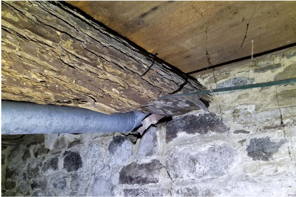
Figure 41: Example of overhead sleeper.
