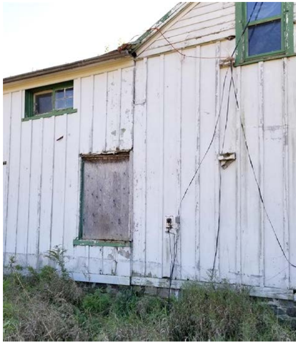
Figure 20: Visible joint between East Wing and Main Block. Note the small horizontal sliding window.
