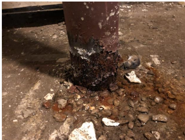
Photo 6- Corrosion at Base of Steel Posts
