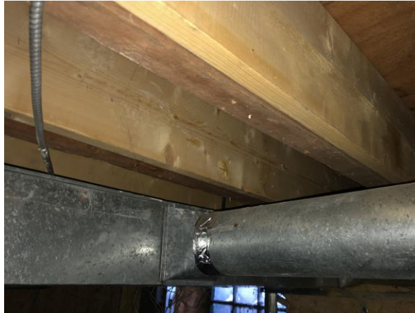
Photo 4- Sistered Basement Joists
