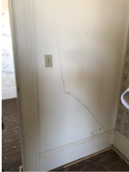
Photo 9- 2 nd Floor Wall Finish Cracking
