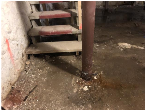
Photo 5- Existing Basement Steel Posts
