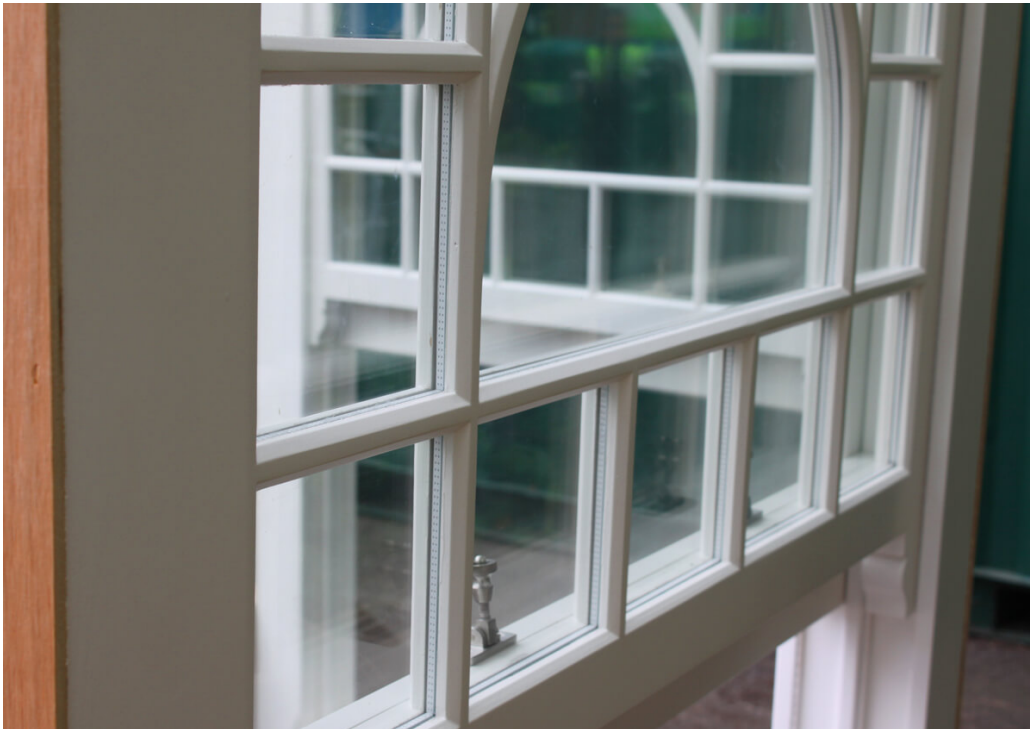
Visual Appearance of Grille Installation
