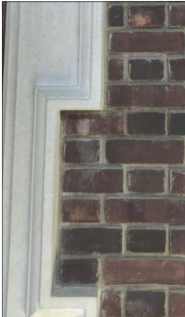
TYPICAL LIMESTONE FINISH PILASTER DETAILS
