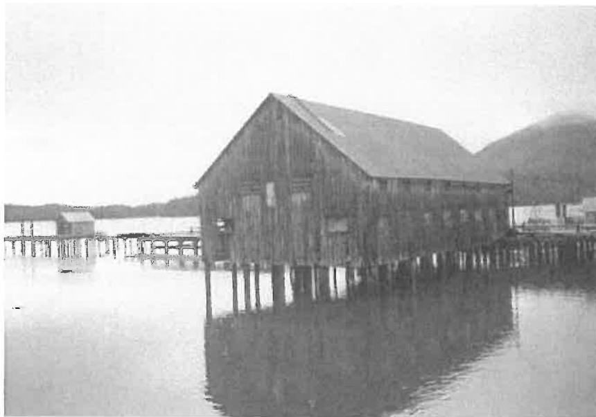
It is important to identify the cause of any damage to a wooden building element before beginning a Preservation treatment. For the former machine shop of the North Pacific Cannery in Port Edward BC, exposure to marine conditions caused the exterior wood cladding to deteriorate.
