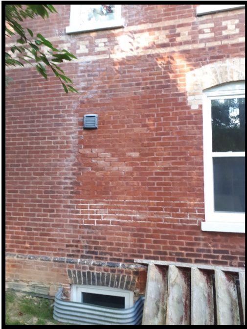
Figures 13 & 14: (Left) View of markings of former addition on the south elevation (Right) Markings on east elevation from former addition (MHBC, 2019)
