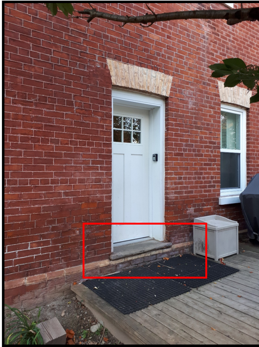
Figure 42: View of rear door opening which will provide passage from the vestibule to the heritage house; red box identifies the wooden threshold of the door opening that may require repair doing new construction (MHBC, 2019)
