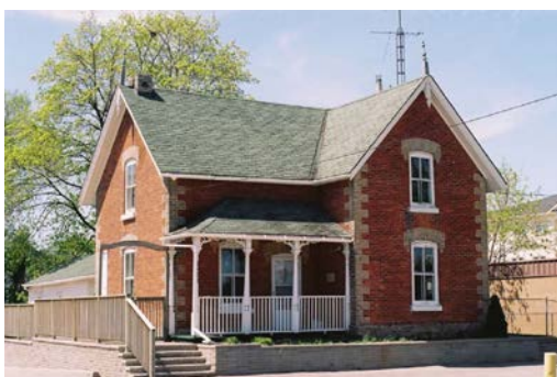
Figure 42 – Brick Quoins on Heritage Structure at 9920 Keele Street , (north of subject properties) from Maple HCD Vol.1
