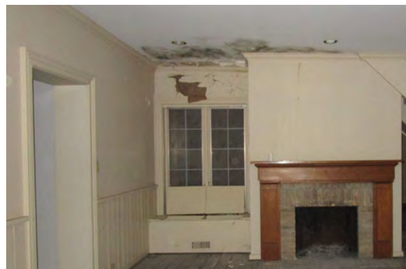
Ground floor interior depicting mould and water damage on wall and ceiling (ERA, 2019).
