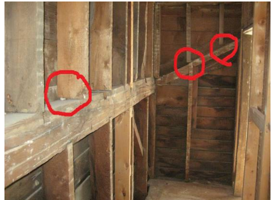
Figure 44. Some of the upper addition studs are not properly seated on the original top plate. My
