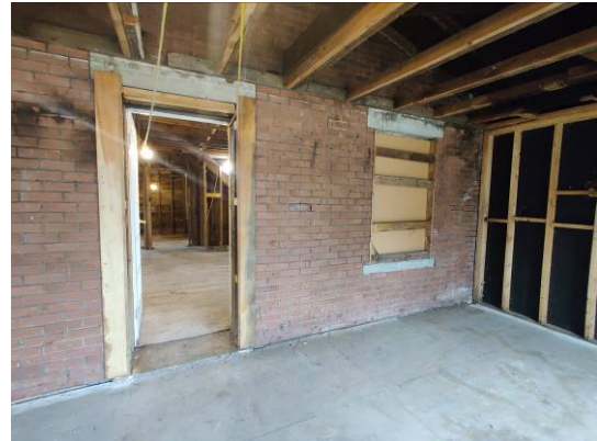
Figure 15. Looking from the verandah into the house.
