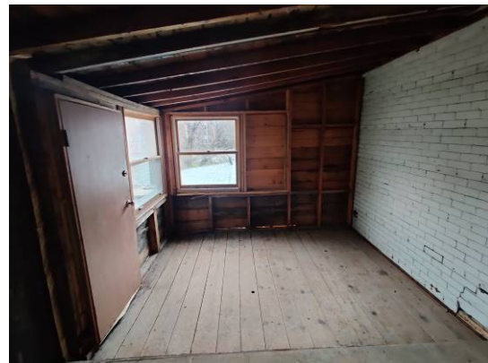
Figure 21. Same room as Figure 20 but looking south.
