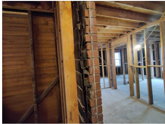
Figure 23. Surprise! Underneath the brick veneer is the previous cladding of untapered clapboard—very much old style.
