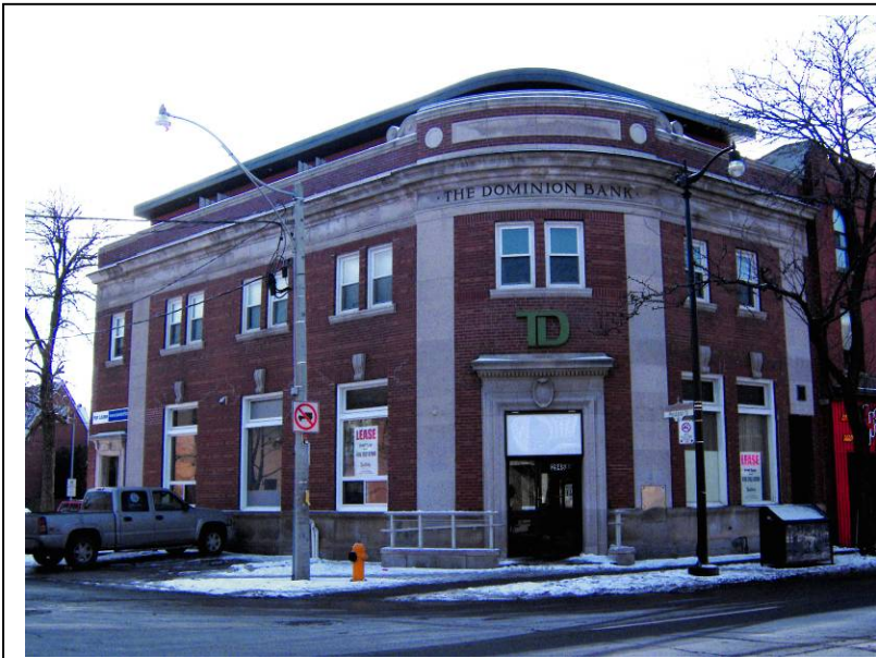
Setting back the third-floor addition allowed the restored bank building to retain its street presence, and maintain the detail significance of the cornice and entry-bay decoration.
