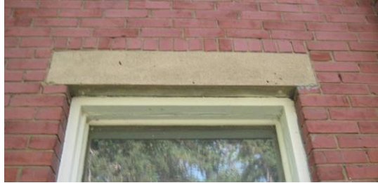
Figure 34. Lintels appear to be of homemade concrete castings rather than limestone or factory precast.
