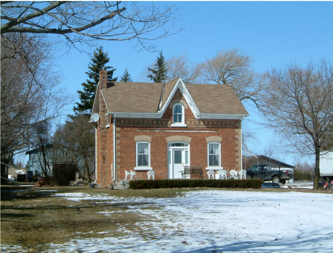
Figure 1. 6120 King Vaughan Road, South Elevation (City of Vaughan 2005).
