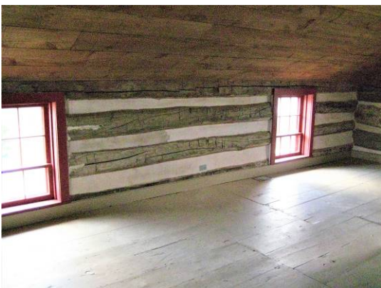
Figure 31. Original house may have had low 2 nd floor windows, as in the Pendergast Log House shown here. Photo by Vic Snow.
