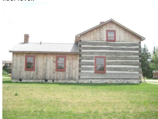
Figure 28. Board and batten kitchen tail of the relocated Pendergast Log House, Brampton. The footprint of the log house is almost identical to that of the original house at 10555 Islington Avenue. This house was also covered in brick in the 1920s. Photo by Vic Snow.
