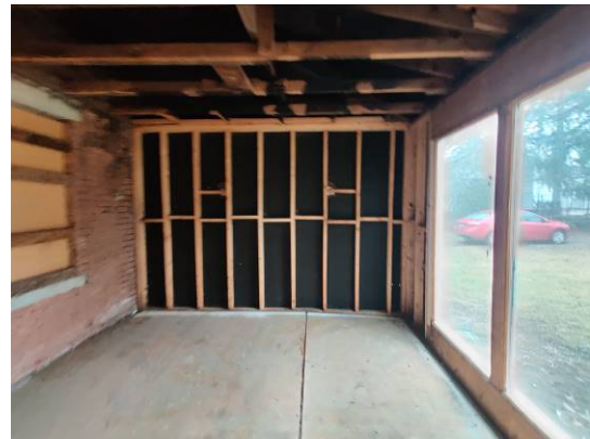
Figure 14. Looking south in the front verandah. Wall construction is relatively recent.
