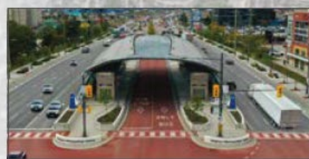
VMC BRT Station
