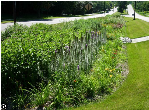
Biofiltration swale/ drainage feature
