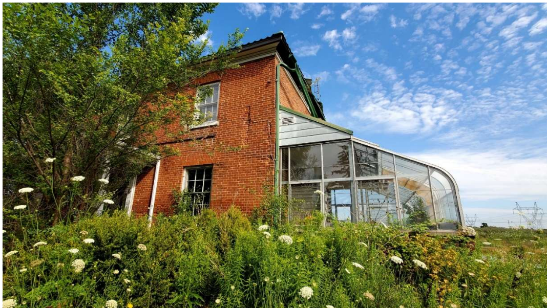
Pic. 4: Southside view showing Greenhouse Addition on Eastside
