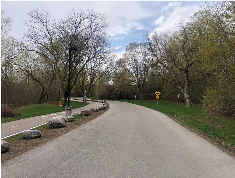
Image 1: View of the driveway at the entrance to the park in the northeast corner of the project area.
