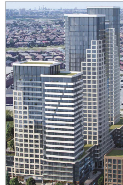
Building C Towers
