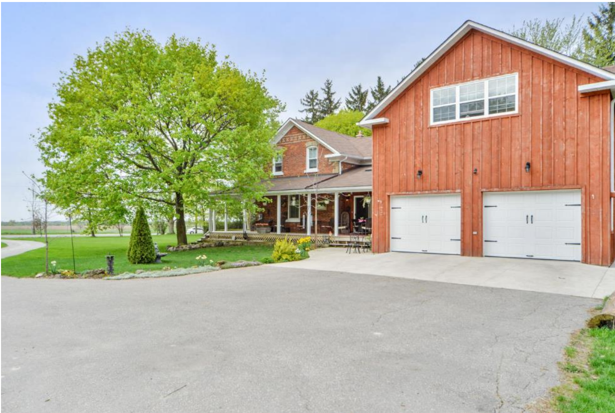
Figure 7. 6120 King Vaughan East Elevation and Addition. (2013 Listing. https://tours.virtualgta.com/public/vtour/display/109751?a=1#!/ )
