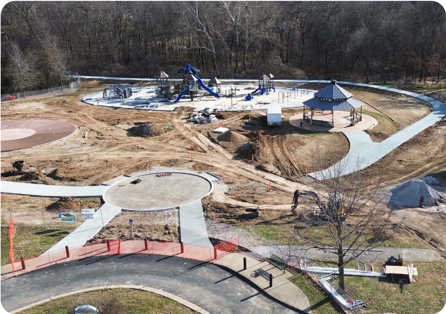
Figure 93 - Millennium Park, Creve Coeur, Missouri
