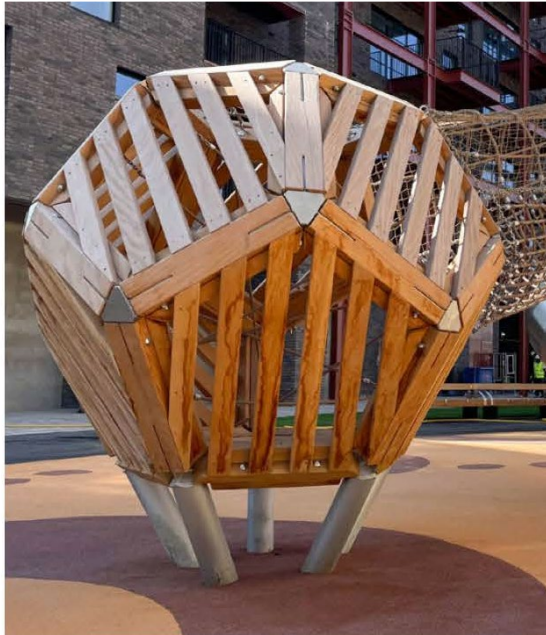
Climber modified to open side with mesh and transfer platform
