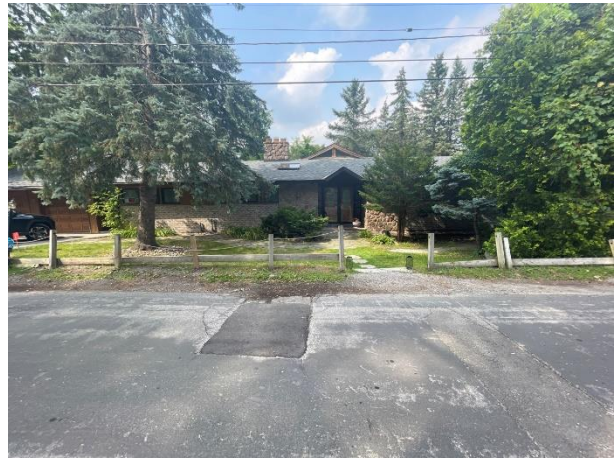
Photo 23 Modernist residence, 18 Mill Street, looking north
