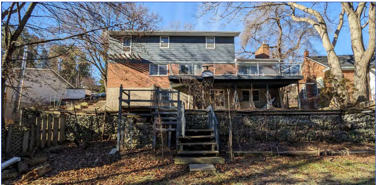
Photo 15: View of the east elevation
