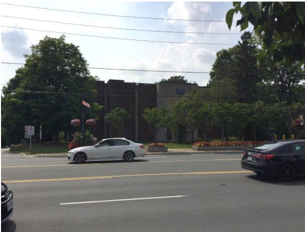
Photo 22 Brutalist structure, 7700 Yonge Street, looking west
