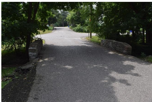
Photo 30 Bridge over creek on Elizabeth Street, looking south
