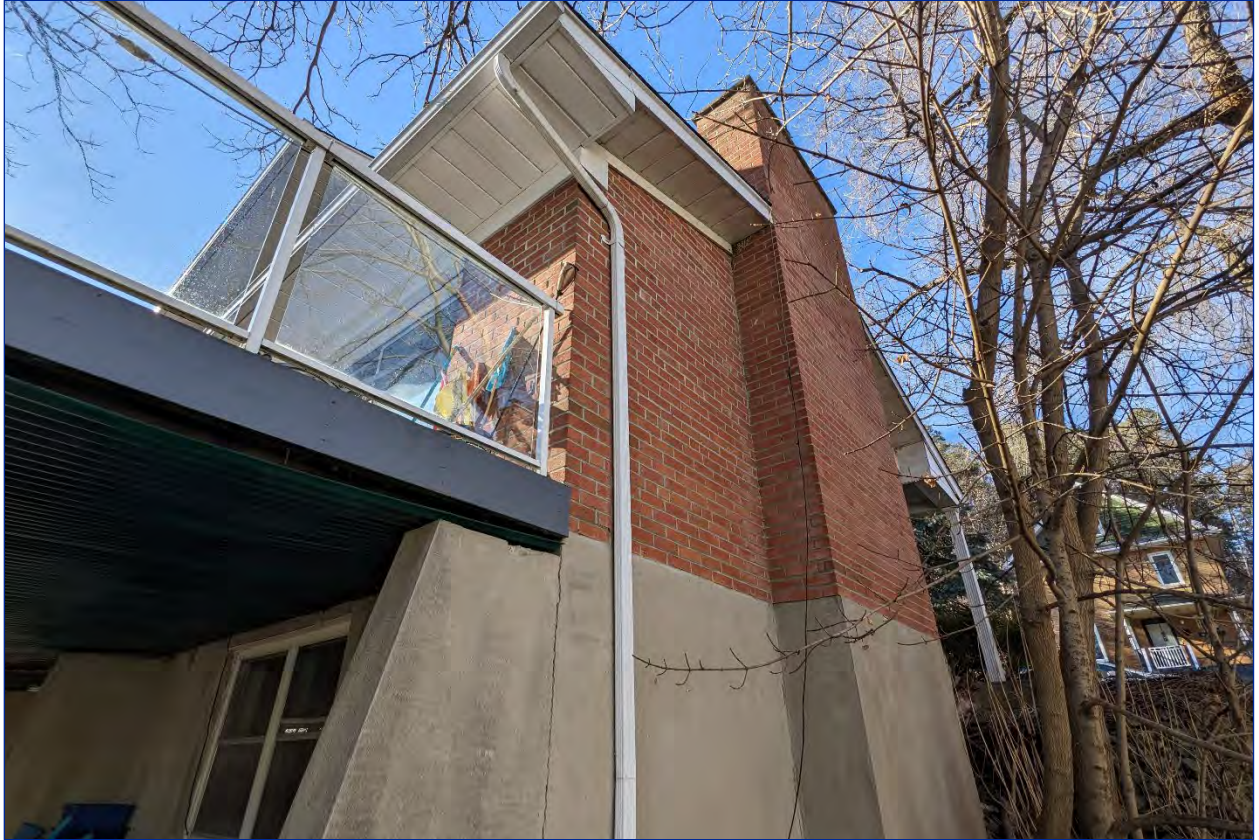
Photo 16: View of the north elevation
