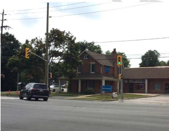
Photo 16 Edwardian influenced residence, 7666 Yonge Street, looking southwest
