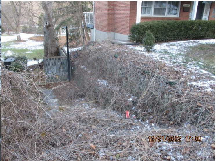
Gabion baskets at front of house
