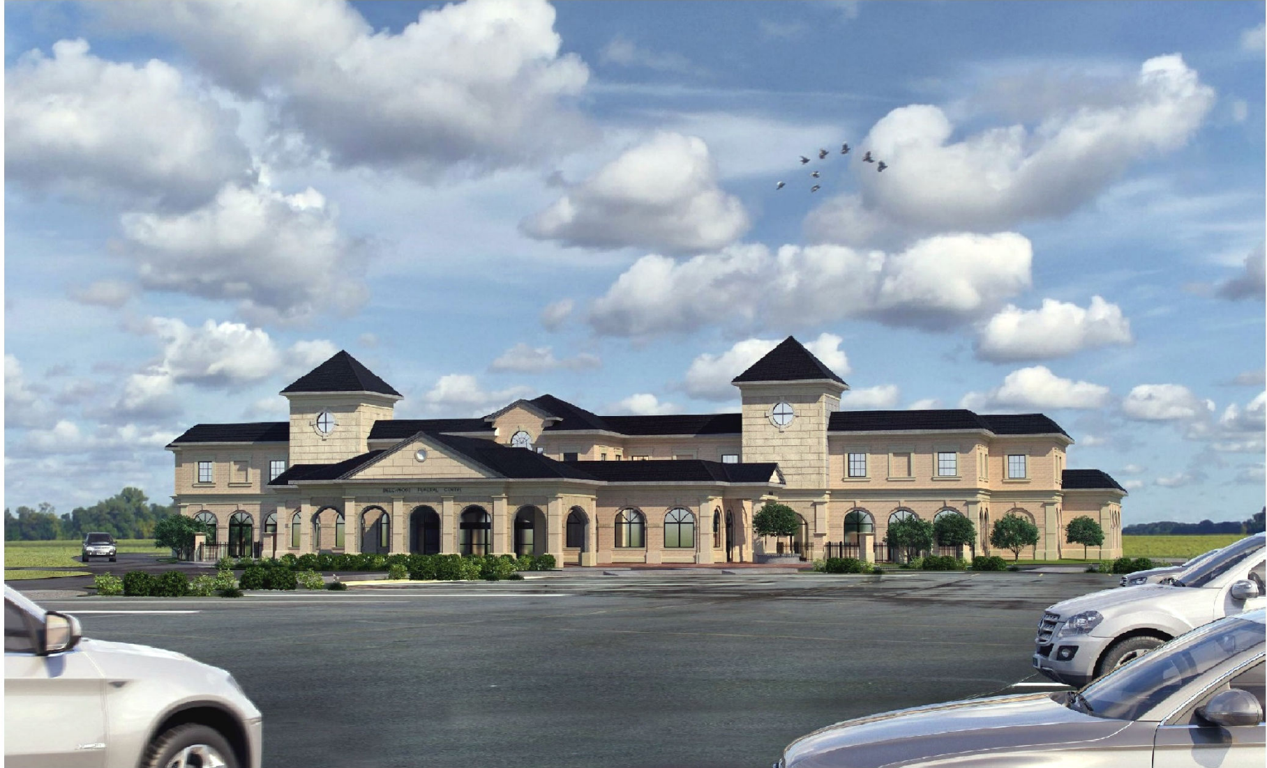
Front Entrance Facing Jane Street
