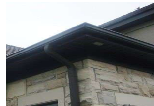
SOFFIT, FASCIA, DOWNSPOUT
